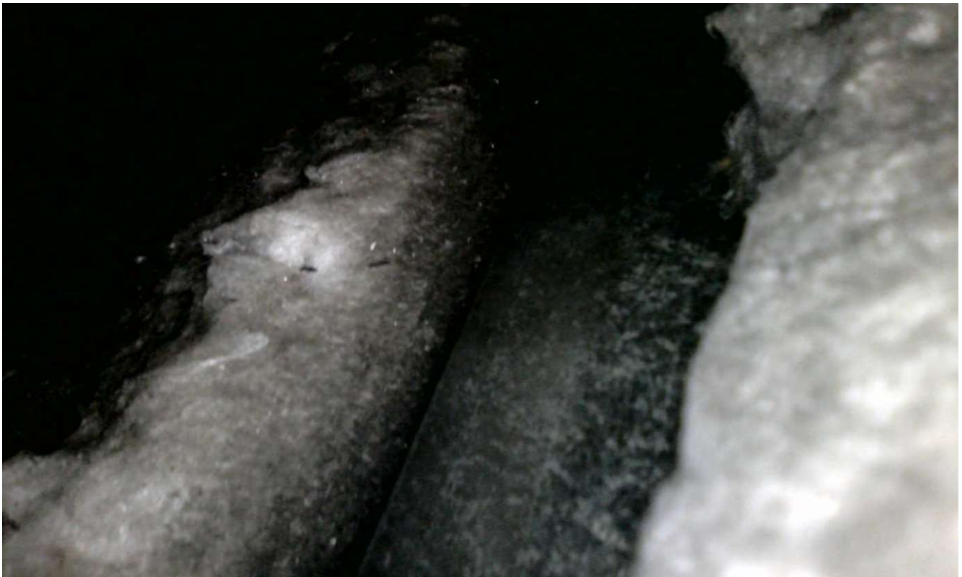
Annex Burn Room Wall Insulation
