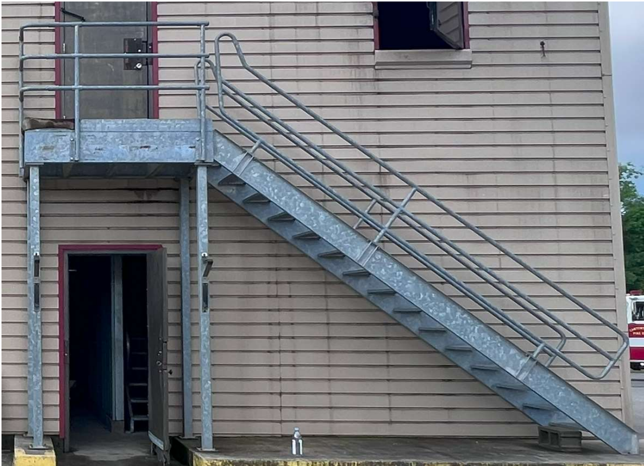
Overall of Hot Dipped Galvanized Exterior Stair Structure
