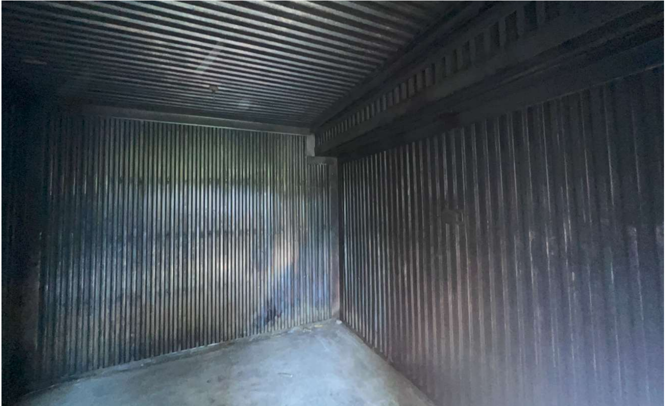
Burn Room #3 Ceiling Panels, Wall Panels & Trims
