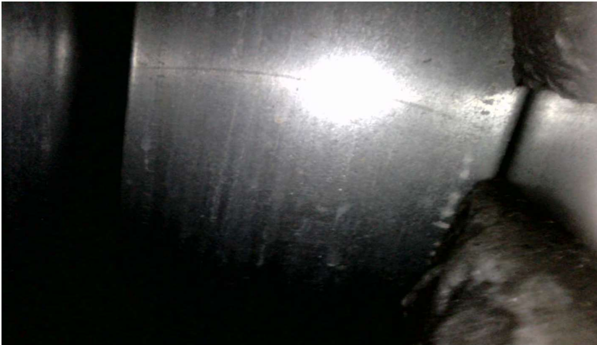
Annex Burn Room – Light Gauge Metal Stud
