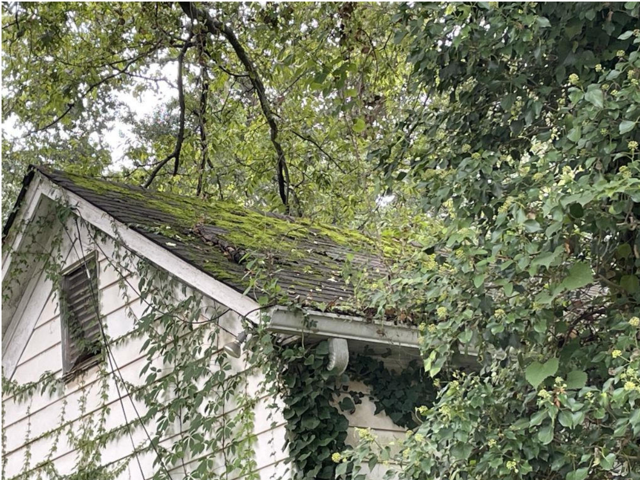
Roof from NE corner.
