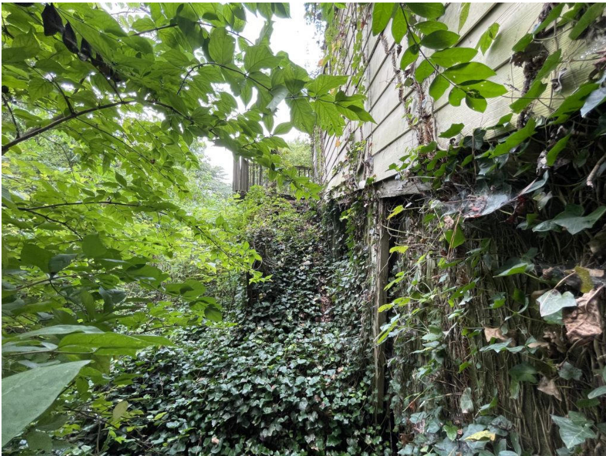
View to rear of home from SW corner
