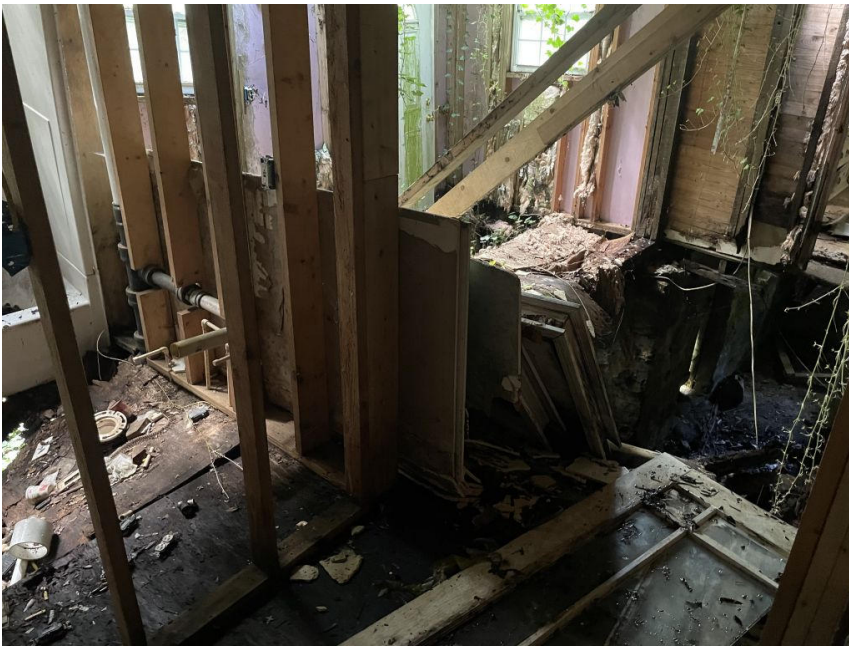
View into addition from Left rear room.
