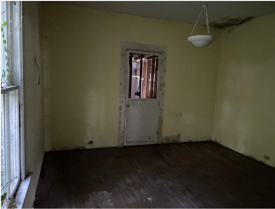
Left rear room abutting addition.
