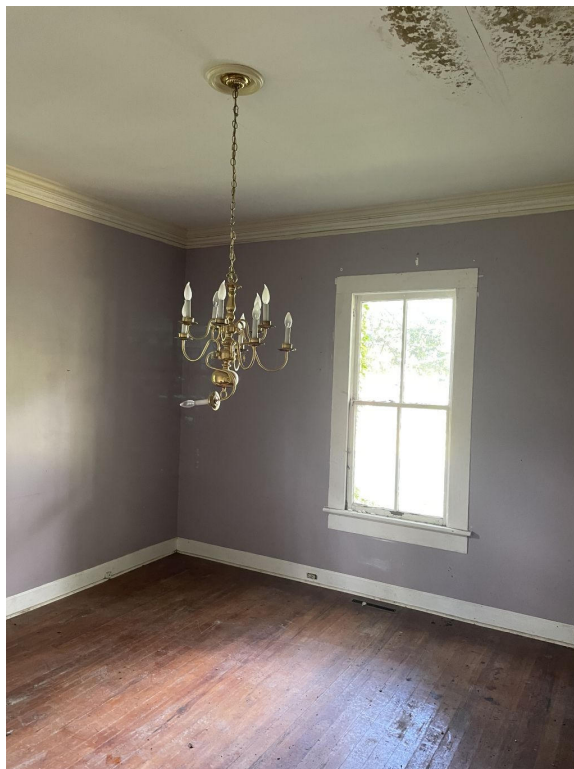
View across Right front room from corner.
