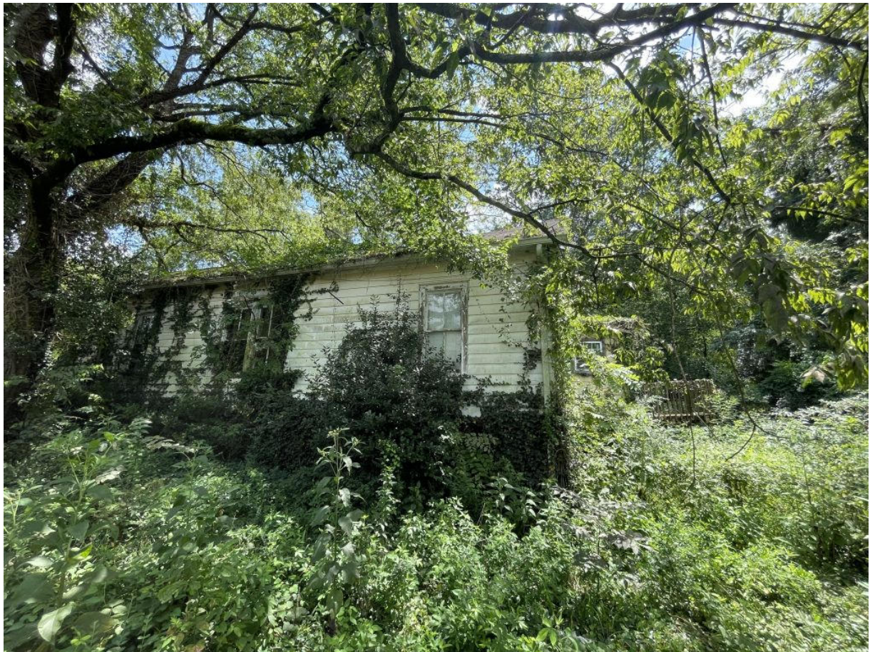
View to northern wall from NW corner
