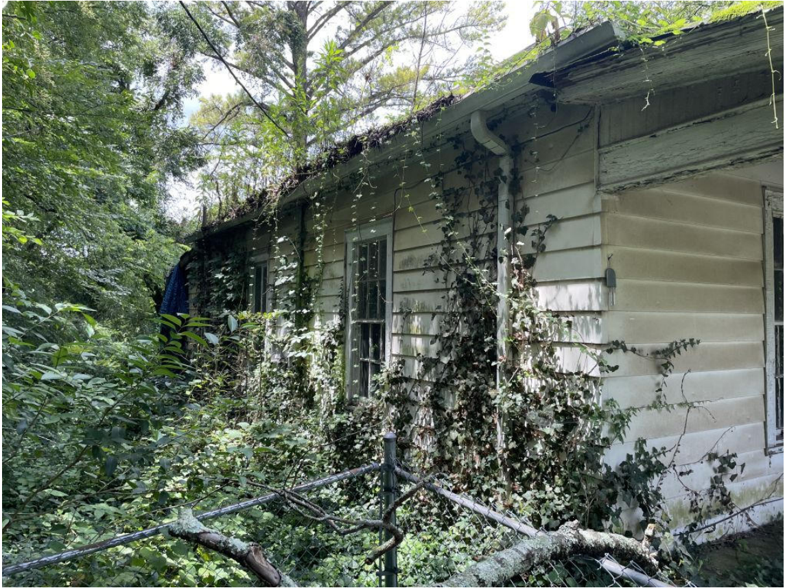
View to south wall from SE corner
