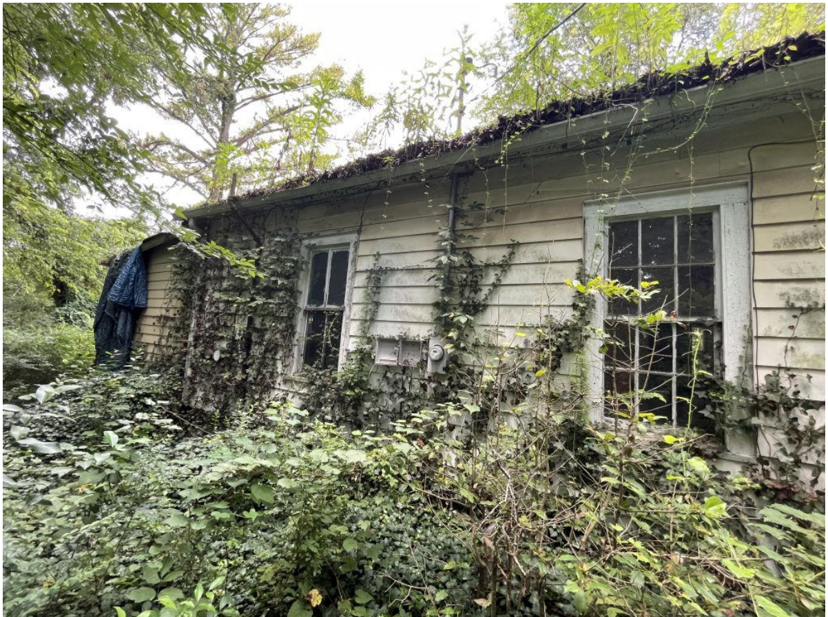
View to south wall from SE corner
