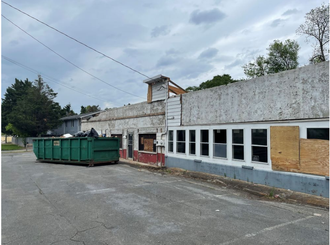
COP22-10. Site Visit on 4-14-23. Interior demolition started.
