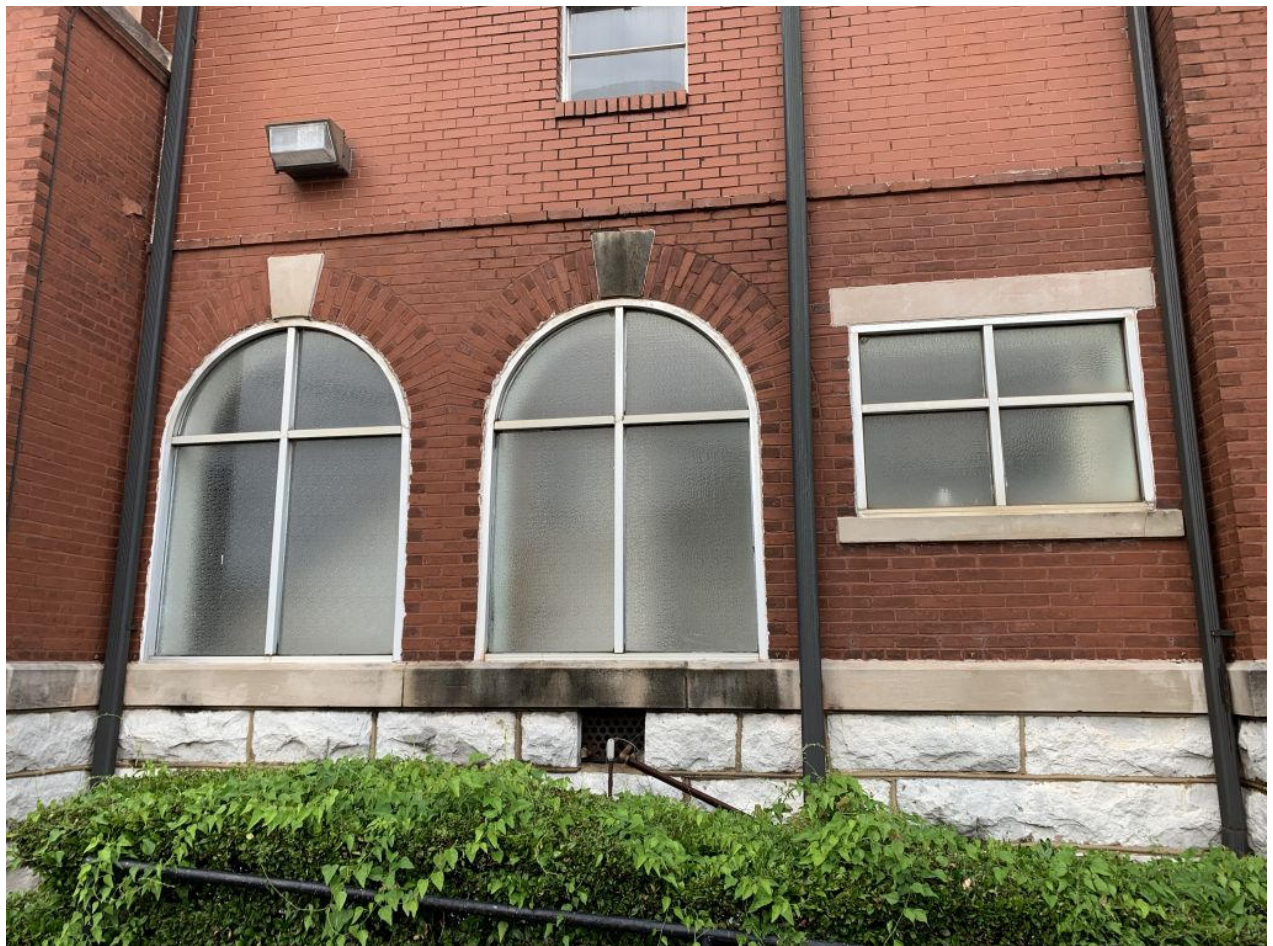
Existing windows appear to be acrylic.
