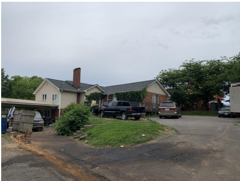
VIEW NORTHWEST TO 1008 STRUCTURE.
