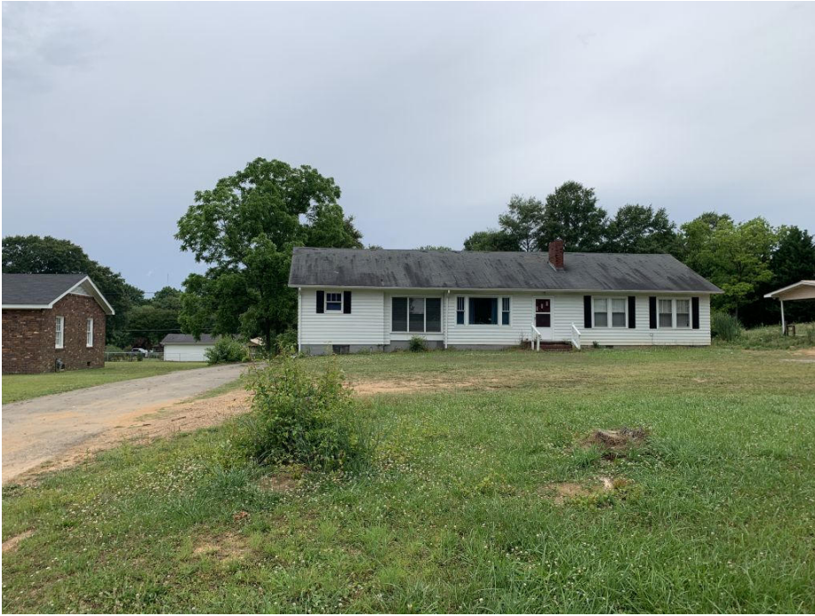
VIEW WEST TO 1006 STRUCTURE.
