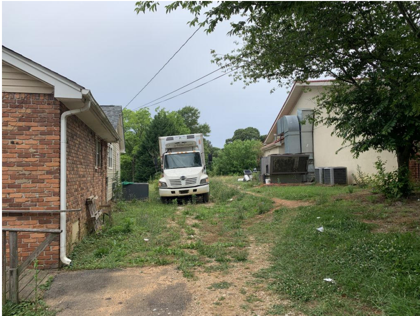
VIEW WEST BETWEEN 1008(LEFT) AND 1010 (RIGHT) STRUCTURES.
