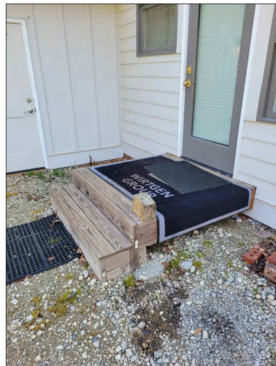
7 OAKLAND STREET BACK DOOR
