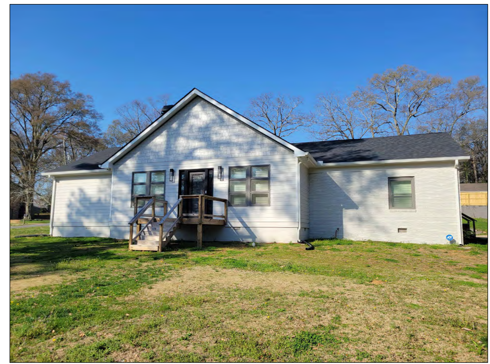
7 OAKLAND STREET EXISTING FRONT VIEW
