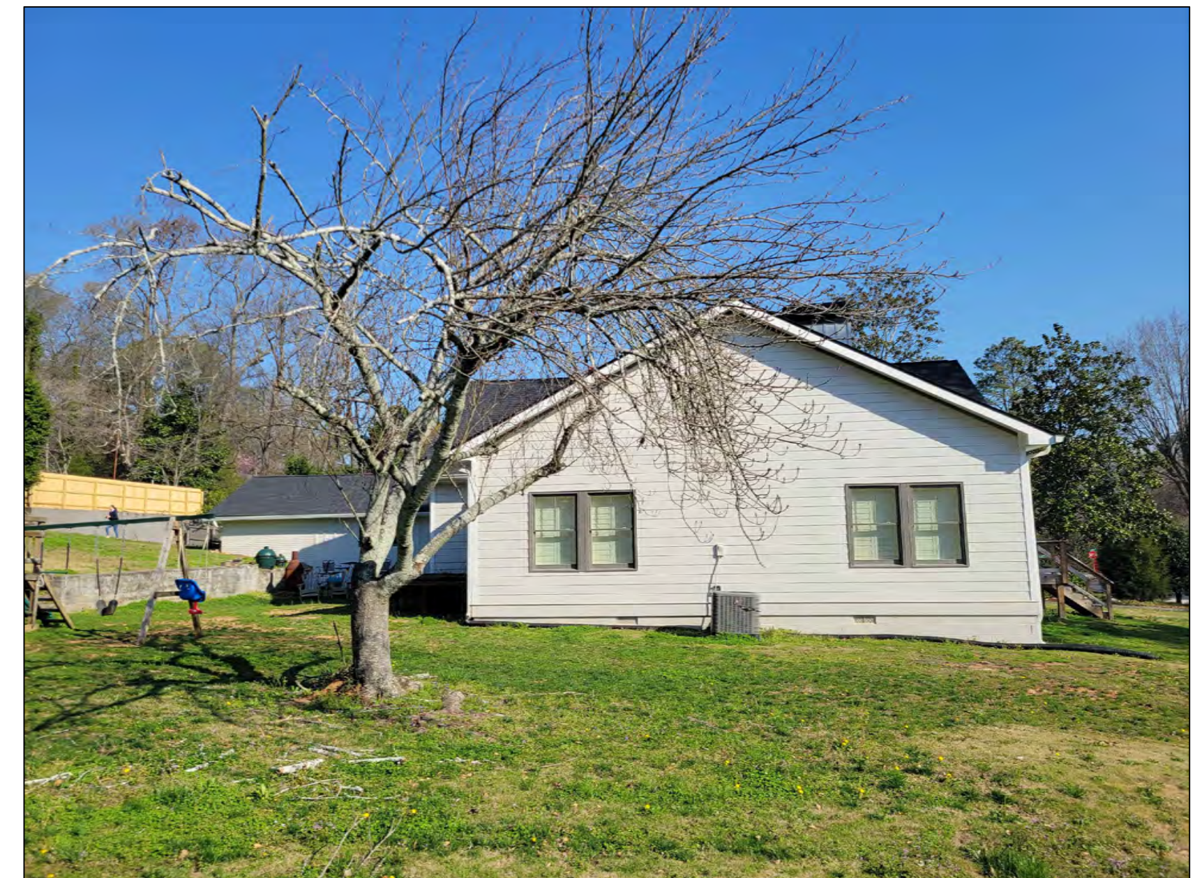
7 OAKLAND STREET EXISTING SIDE VIEW - POPLAR STREET
