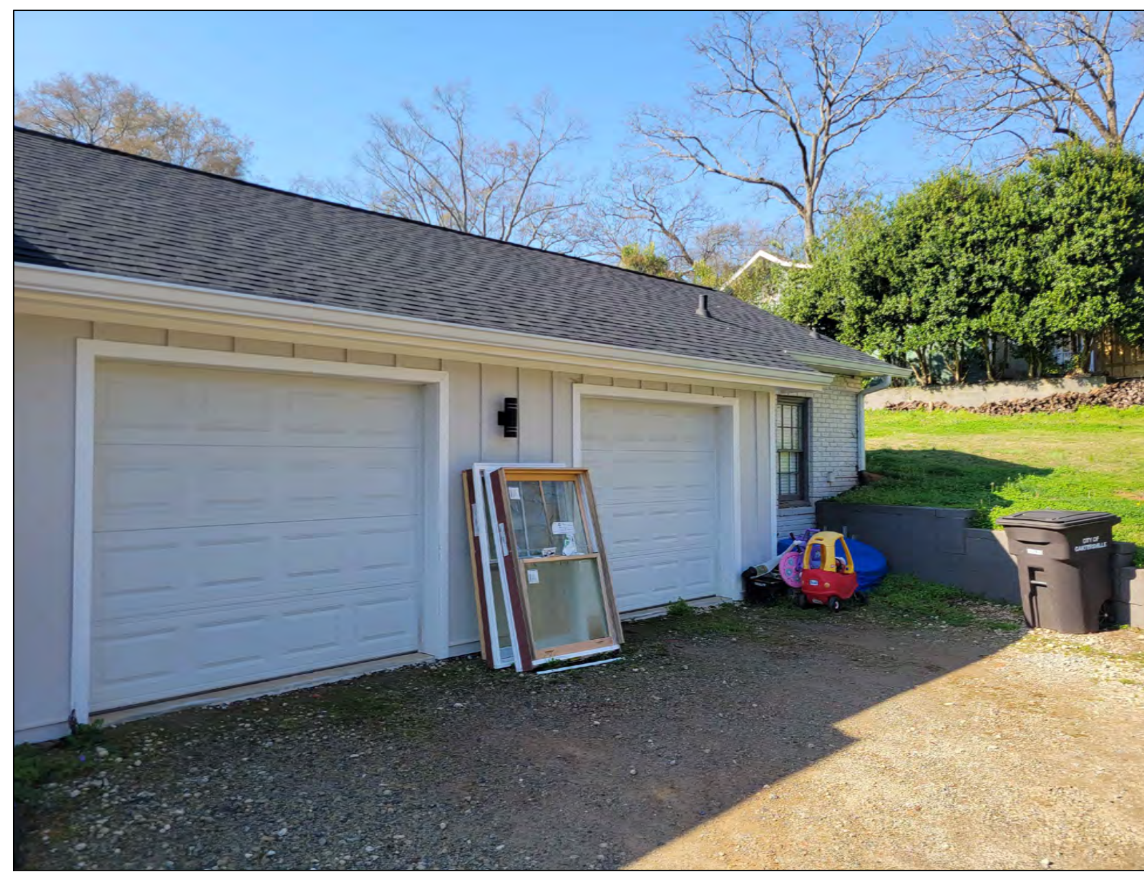
7 OAKLAND STREET EXISTING GARAGE VIEW
