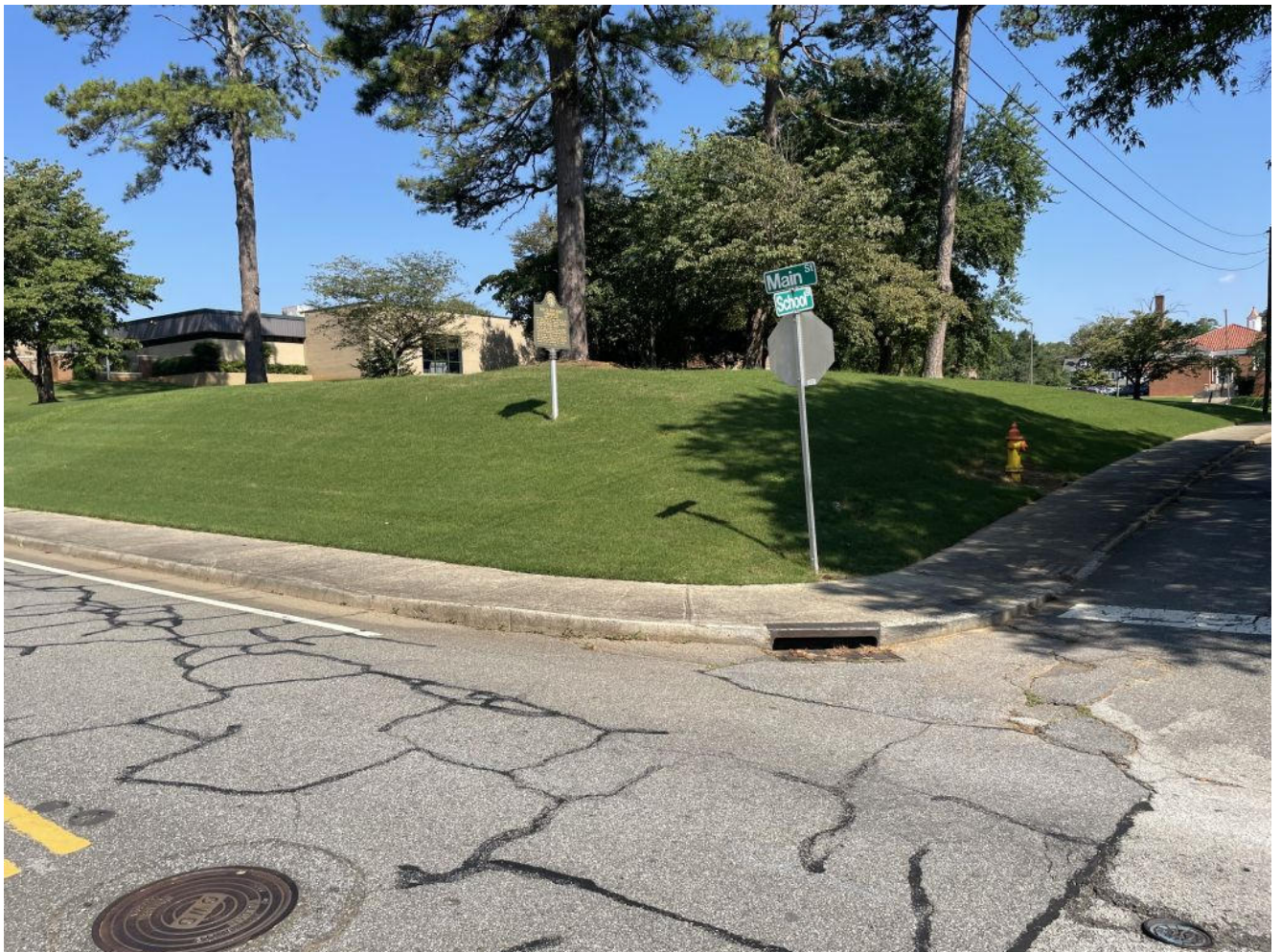
View West along W. Main St. at School St.
