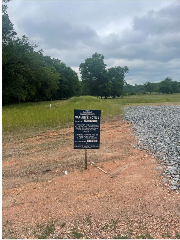
Cass- White Rd Construction Entrance
