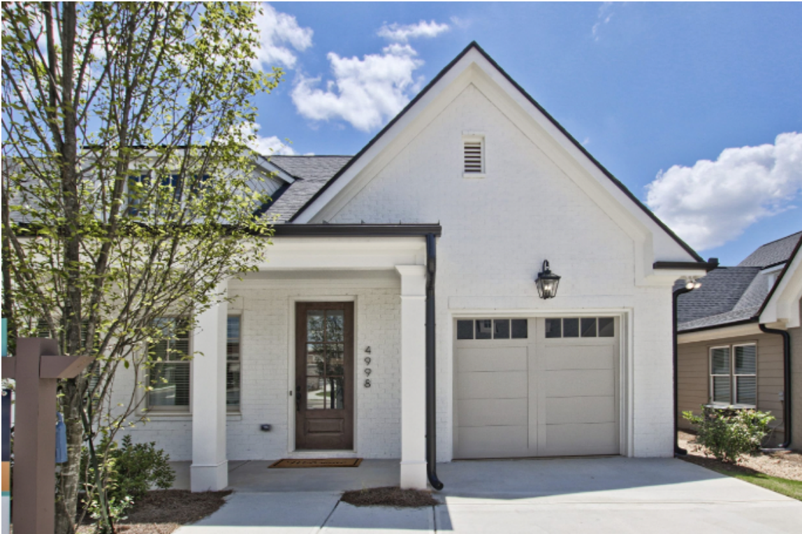
RIGHT SIDE OF "EVERGREEN" UNIT
