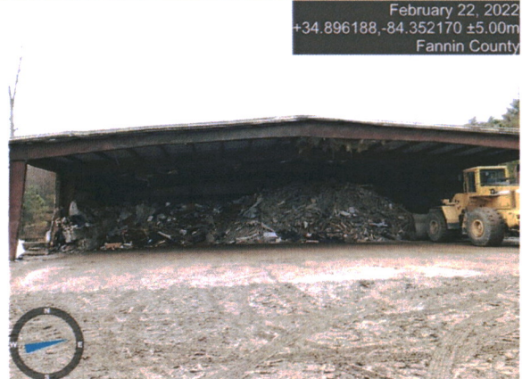
Photo Number: 2 of 4 Date: 2/22/2022 Time: 11:00 AM Weather: overcast Location: Sugar Creek C&D Transfer Station County: Fannin Photographer: Jason Rogers Observations: Front view of transfer station, showing no partitioning between municipal waste (left side) and C&D waste (right side)
