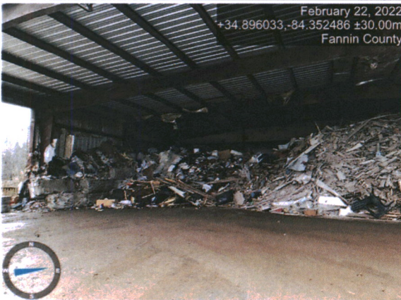
Photo Number: 3 of 4 Date: 2/22/2022 Time: 11:00 AM Weather: overcast Location: Sugar Creek C&D Transfer Station County: Fannin Photographer: Jason Rogers Observations: No partitioning between municipal waste (left side) and C&D waste (right side)
