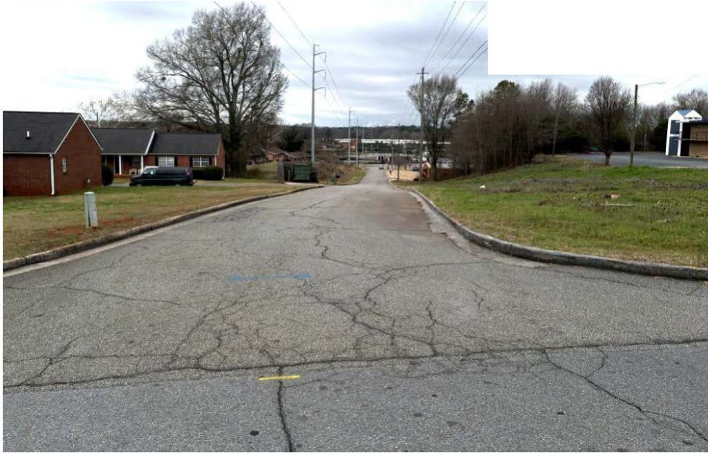
View west along Brook Dr from SE corner of project site. Paladius duplexes on left.
