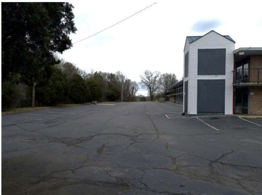
SW corner of project site. View north along hotel rooms.
