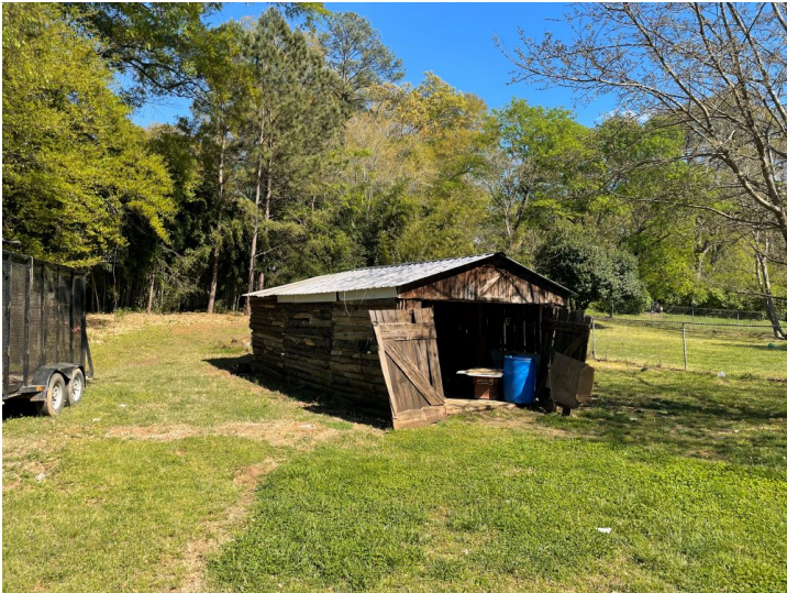
Storage shed to be demolished
