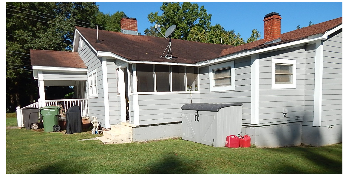
BACK CORNER VIEW
