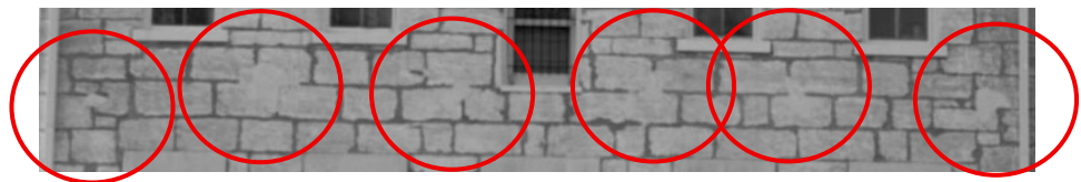
Close up of THC 1969 Survey photo of south elevation, possible stone patchwork
