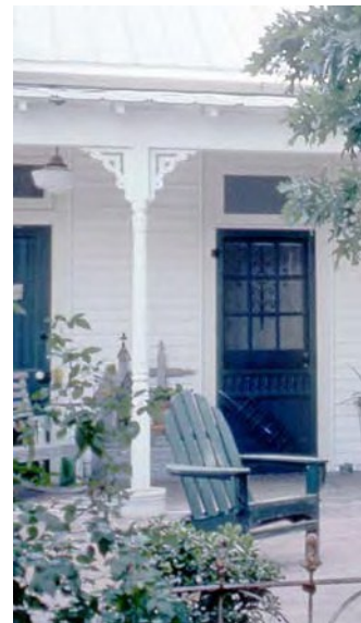
Columns with fan brackets
