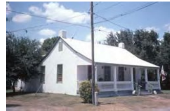
Many stone houses were covered with protective limestone plaster or stucco painted white or cream color.
