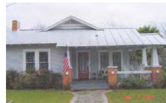
Brick column base is typical on bungalows with "missing" upper part of column
