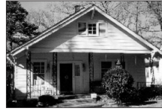
Restoration of original porch columns is encouraged. Replacing the "licorice stick" wrought iron columns used here with columns like these restores the building appropriately.
