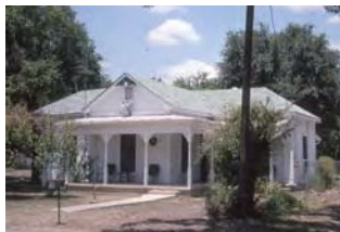
Combination Hip Roof
