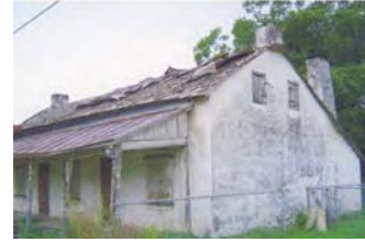
309 Paris. Original cypress shingles were often covered over with a metal roof, leaving the shingles in place
