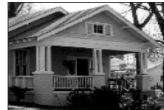
Restoration of original porch columns is encouraged. Replacing the "licorice stick" wrought iron columns used here with columns like these restores the building appropriately.
