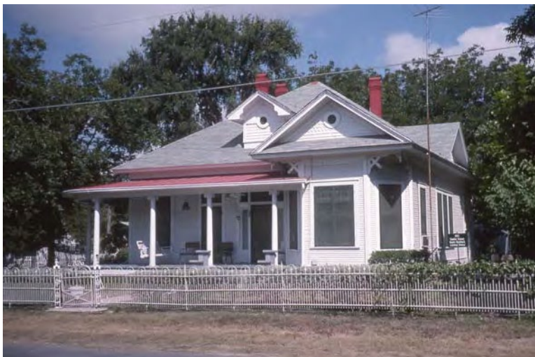
Some houses have decorative “fish scale” shingles, as well as regular shingles and horizontal siding.
