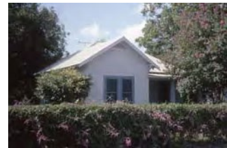
Later 19 th century houses used horizontal wood siding, which should be regularly painted.
