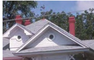
Soffits on Gable End and on Dormer
