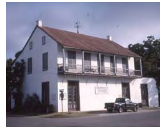
Two-story porch without column supports at the ground level.
