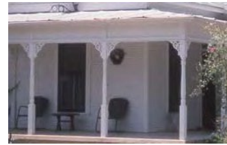
Columns with fan brackets
