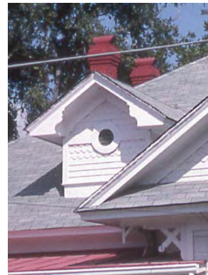
Boxed eaves, wheel window, and corbelled chimney caps
