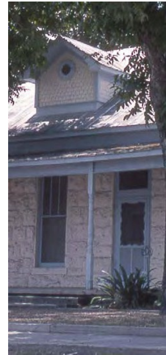
"Fish scale" shingles on the dormer and decorative screens are important details on this house.
