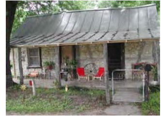
Wood frame and infill stone
