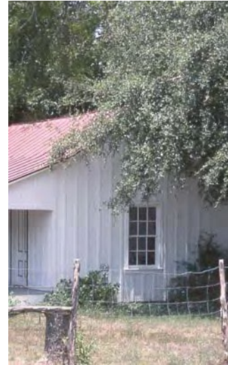
An example of board and batten siding.
