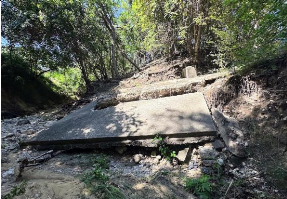
1 – Structural failure of the side channel concrete apron due to scour-induced undermining. (Facing downstream)
