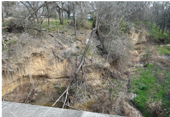
4b – Overhanging bank condition caused by toe erosion resulting in bank collapse, vertical banks (~15 ft. height) and mass wasting. (Facing downstream)
