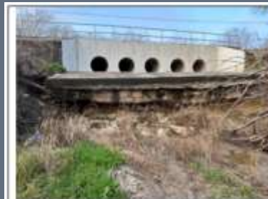
5a – Geneva Street culvert showing scour erosion, undermining of the concrete apron to a cantilevered condition, exposure of water line, accelerated failure of the northern bank. (Facing upstream)
