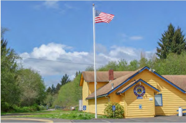
Existing Lions Club building next to Lions Park (Source: Stantec)
