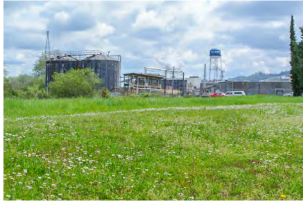
Undeveloped property adjacent to the Cosmo Specialty Fibers mill operations (Source: Stantec)
