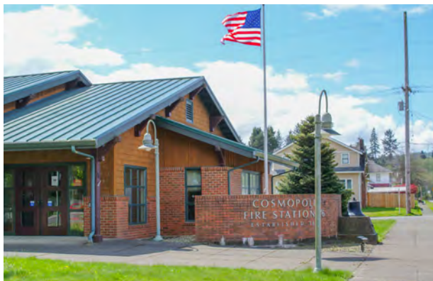
Existing Fire Station building (Source: Stantec)
