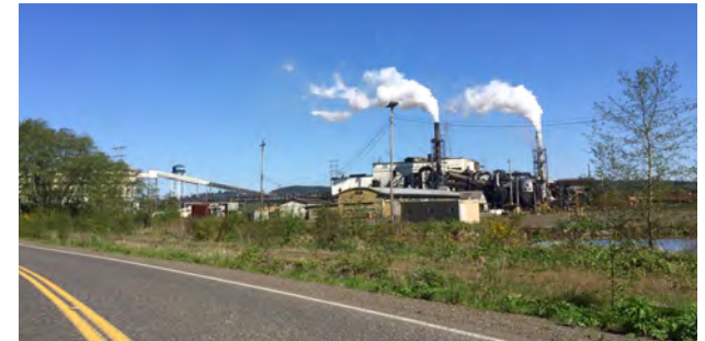
Cosmo Specialty Fibers mill facility (Source: Stantec)
