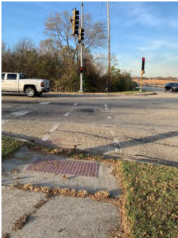
Photo 4 – Looking north at the intersection of Theodore St and Gaylord Rd/Cedarwood Dr
