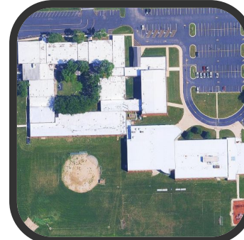
Multi-Million Roof Repairs
