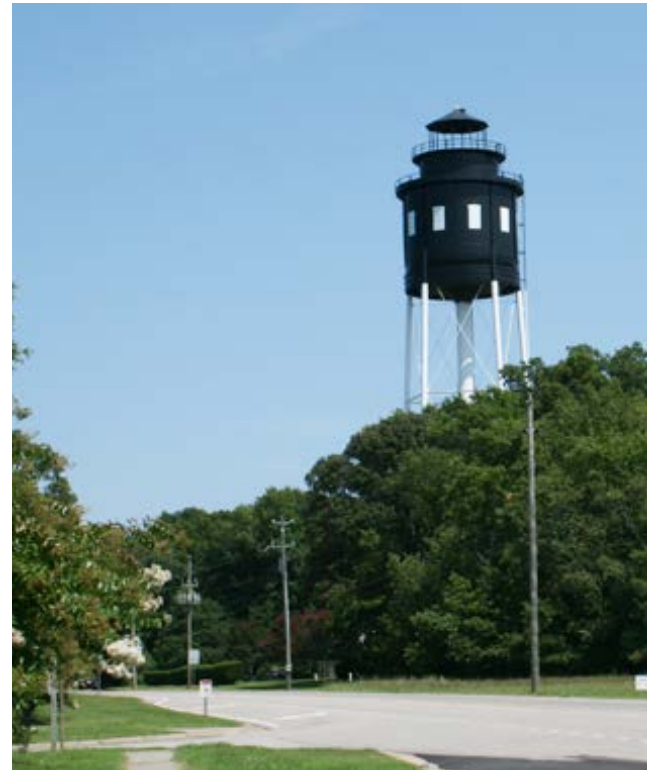
Cape Charles water tower.
