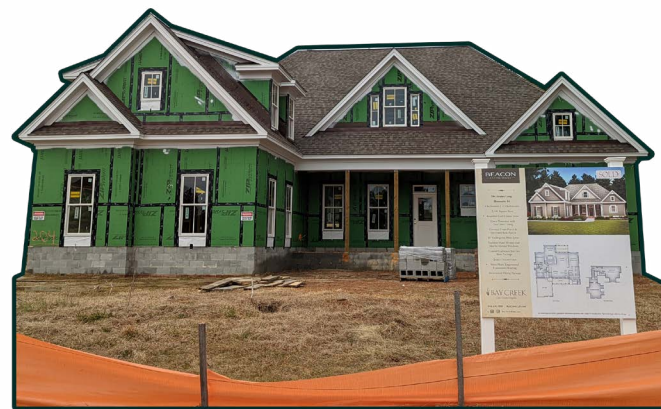
Home under construction in Bay Creek.
