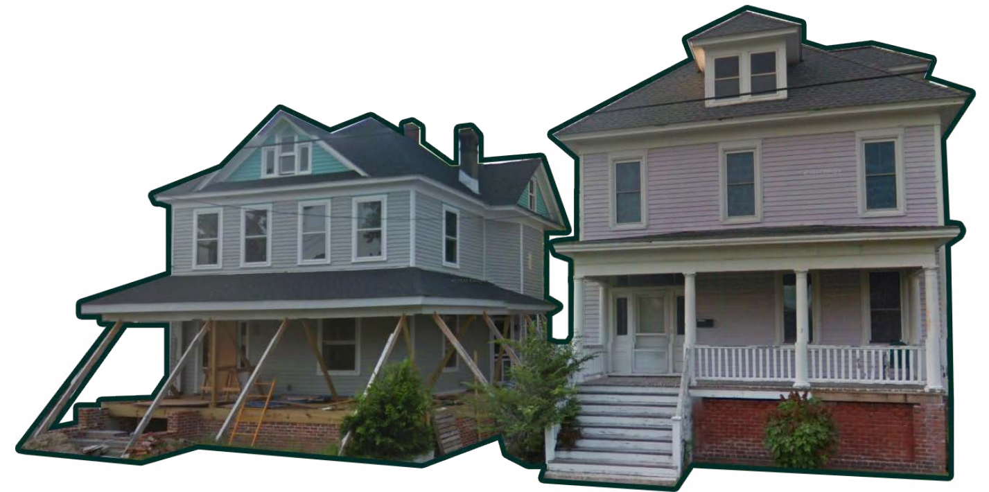
House Renovation in Cape Charles Historic District, Google Streetview
