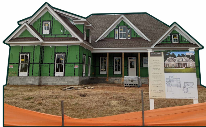
Home under construction in Bay Creek.
