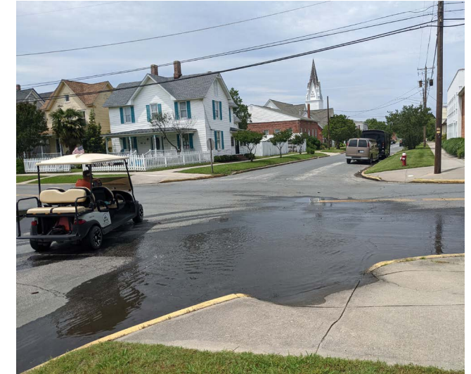
Storm water at Randolph Ave & Plum St intersection.
