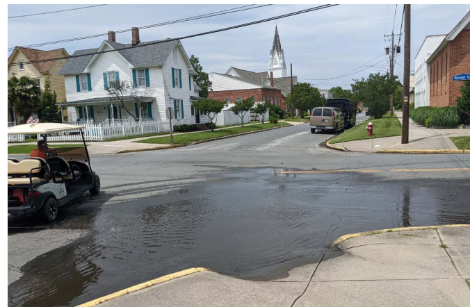
A golf cart drives past pooled stormwater.
