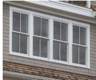
WINDOWS: MARVIN ULTIMATE DOUBLE HUNG ALUMINUM CLAD WITH SIMULATED DIVIDED LITES 2'-2" X 3'- 8" 2 LITES HIGH/ 2 LITES WIDE 2'-10" X 5'-8" 2 LITES HIGH/ 2 LITES WIDE
