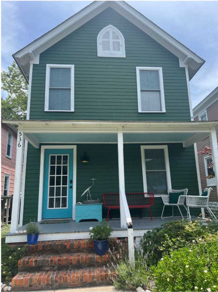
536 Randolph Avenue Existing Conditions
