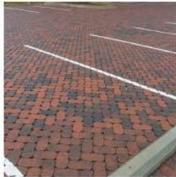
Permeable brick paving
