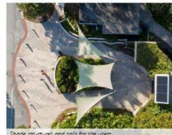
Shade structures and sails for site users.
