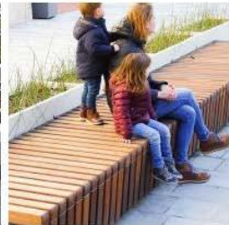
Wood slat benches integrated into seat wall
