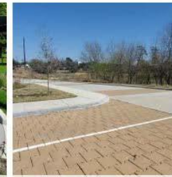
Pavers used for parking bays
