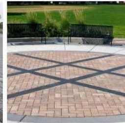
Unique paving pattern at plazas
