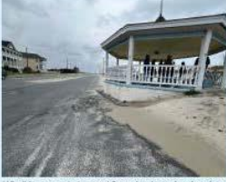
Windblown sand, the sand from the dunes is migrating past the Gazebo and into the road.
