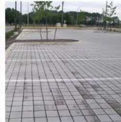
Permeable parking in parking lot
