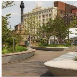
Cast in place concrete seat walls
