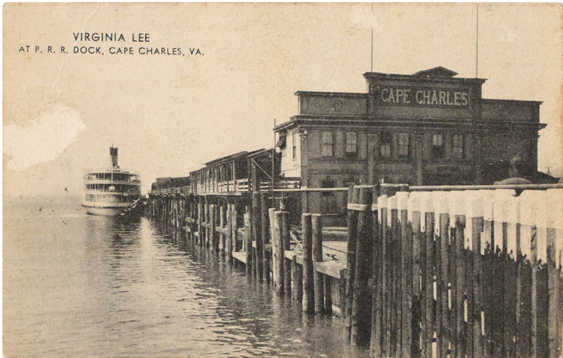
Image 8: Cape Charles harbor and terminal building, 1930.
