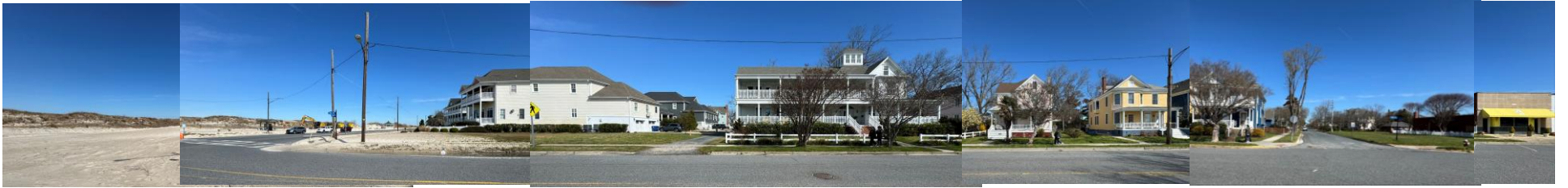
1. Mason Avenue, south elevation, between Bay Avenue and Harbor Avenue
