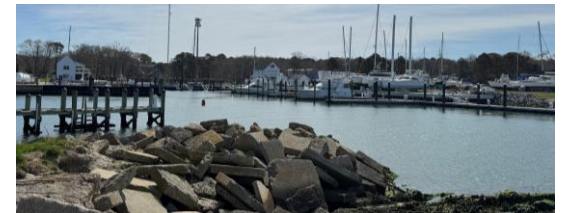
View facing south side
