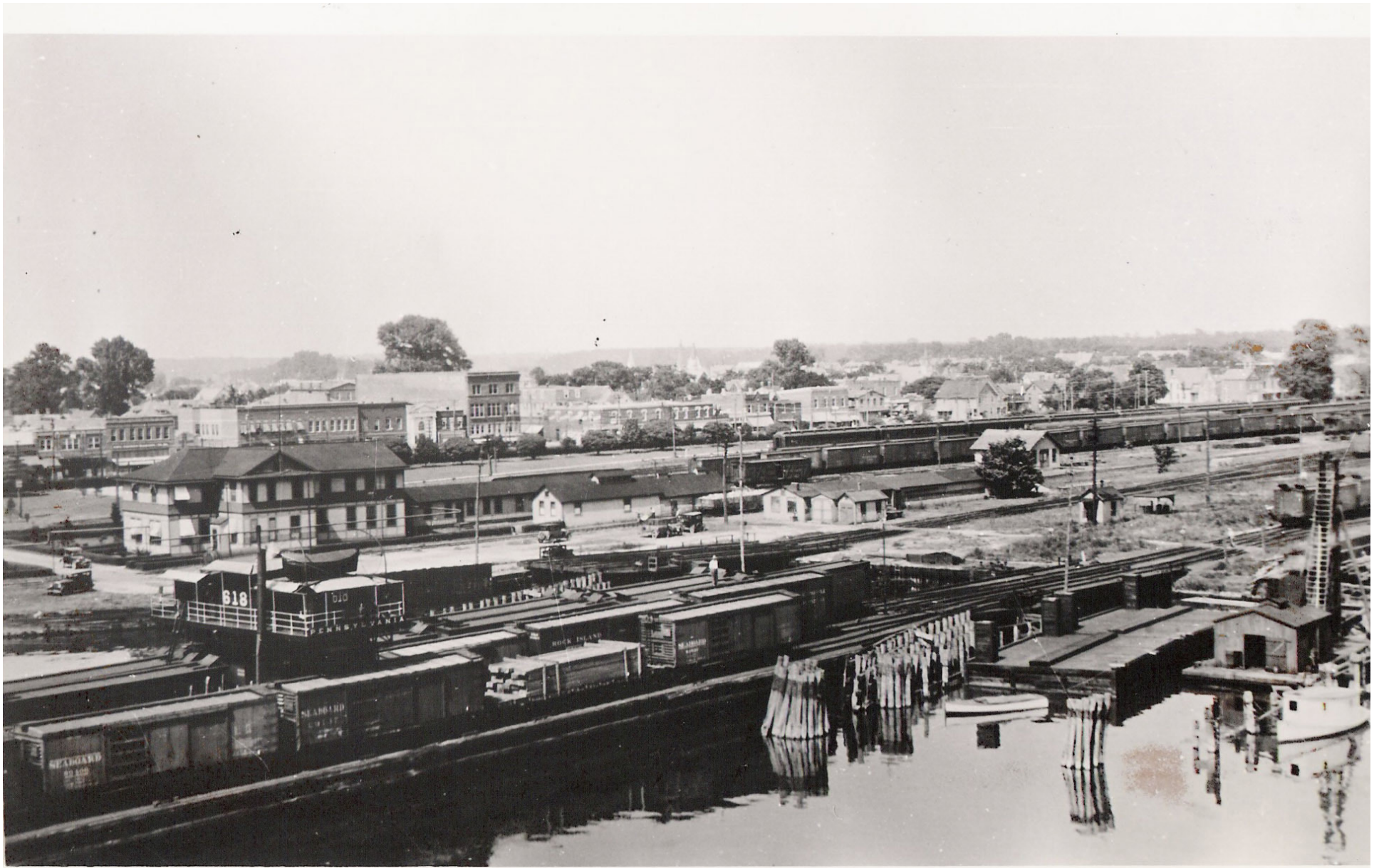
Image 12: Cape Charles Harbor and Railway, 1927. This view, looking east from the harbor, shows more of the Master Plan area, with Mason Avenue, green space, railways, and the harbor are all visible
