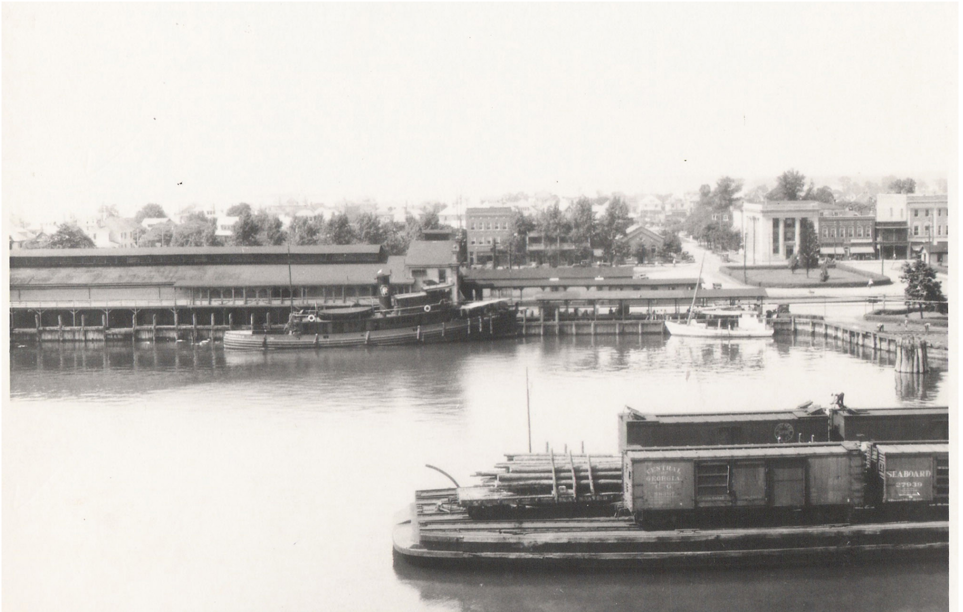
Image 2: Cape Charles Harbor and Mason Avenue 1927. This view provides insight into the historic flow from the town across Mason Ave and into the railyard/harbor area. Public space extending from Pine Avenue functioned as a central axis. The axis and associated public parks and open spaces provided viewsheds and pedestrian access, with industrial-related structures built up along the harbor to the west, and along the railway to the east (see images 1, 5, and 11).
