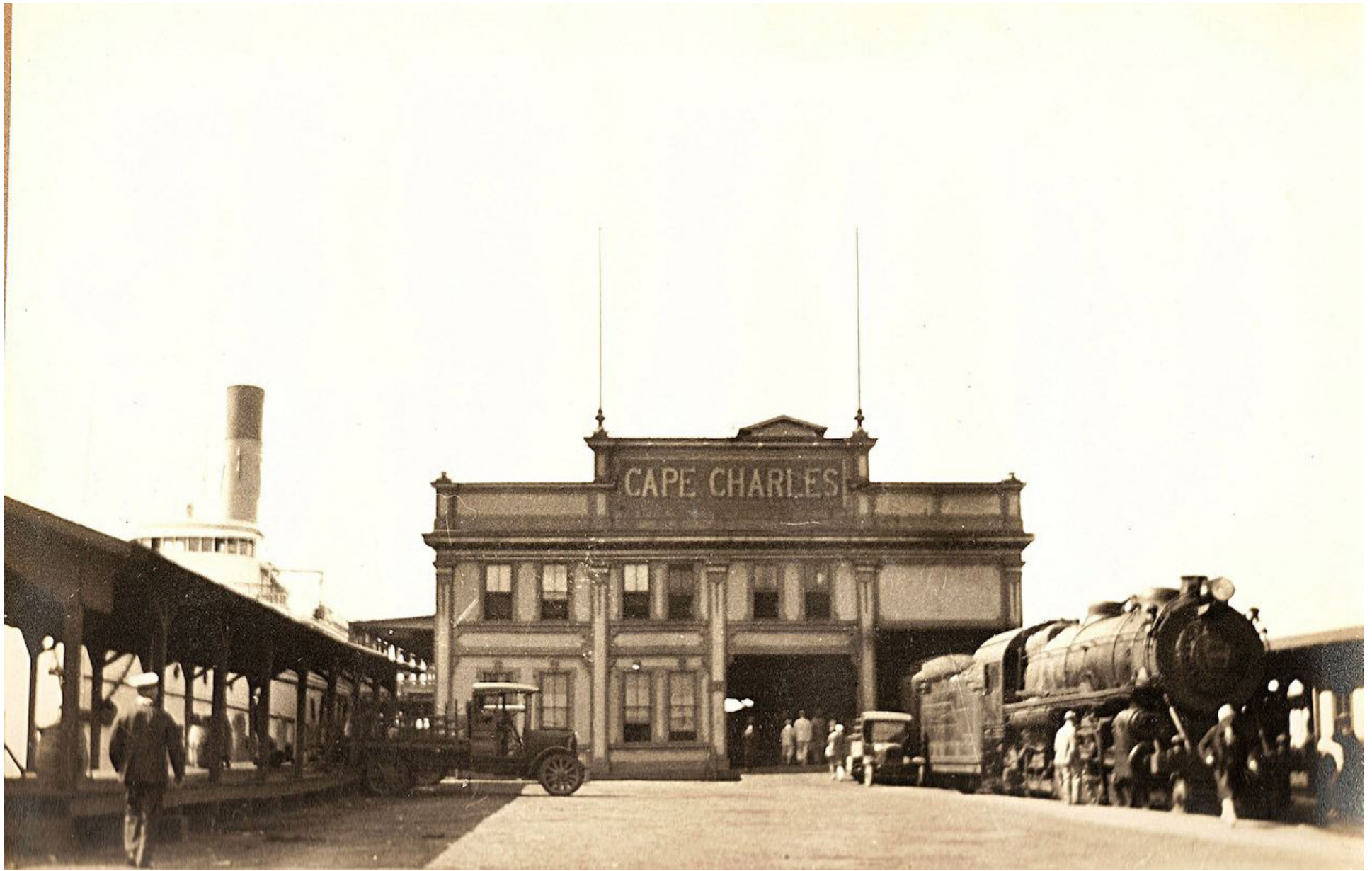
Image 7: Cape Charles Harbor and Terminal Building, date unknown. The Cape Charles terminal building was formidable with a careful design that highlighted the status of the town and functioned as the hub for the center of the town's economy, connecting rail and ferry transportation. This architecture, and other historic architecture associated with the harbor and railway, while no longer extant, may help give a vision of the character of the town historically and how future development and planning can honor or reference that history. The terminal building is also visible in images 1, 4, and 5.
