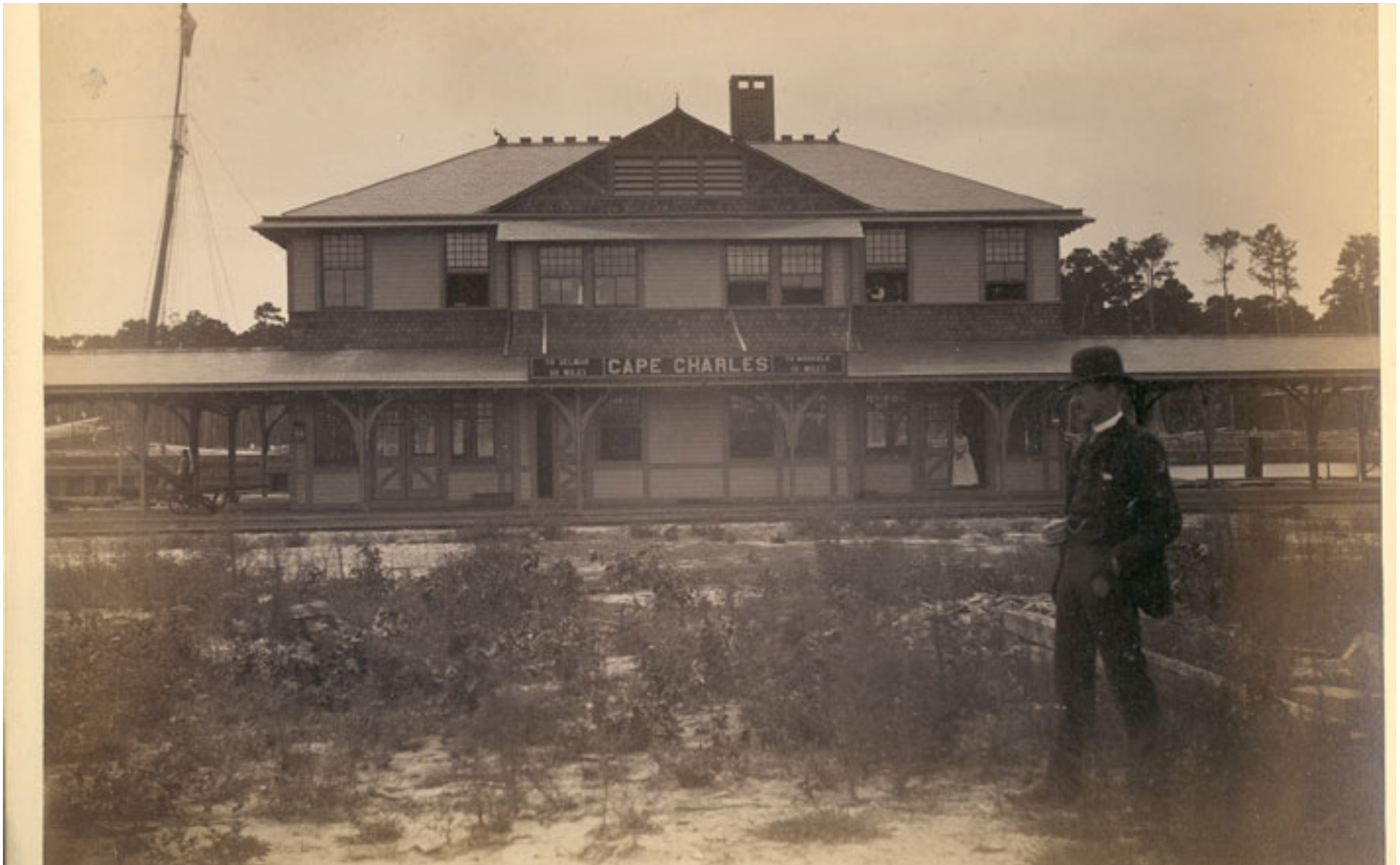
Image 10: Cape Charles Passenger Station, 1885. As with the Harbor Terminal building, the Passenger Station was central to the primary economy of the Town. This building was located east of the harbor terminal building, slightly inland along the tracks from the harbor.
