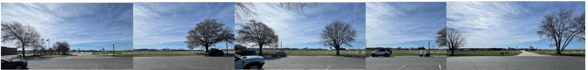
4. Mason Avenue, north elevation, between Pine Street and Harbor Avenue
