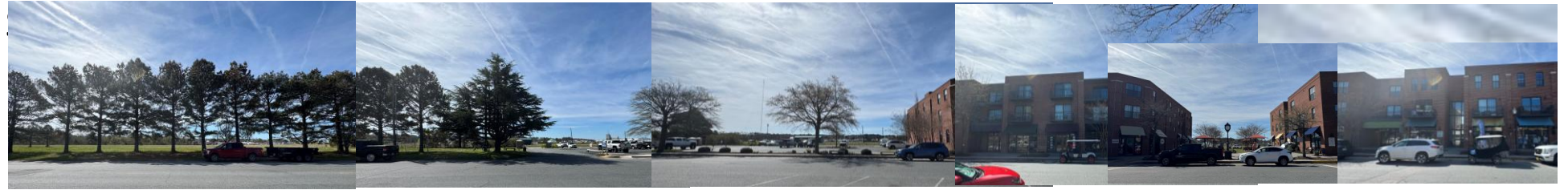
2. Mason Avenue, north elevation, between Peach and Strawberry Streets
