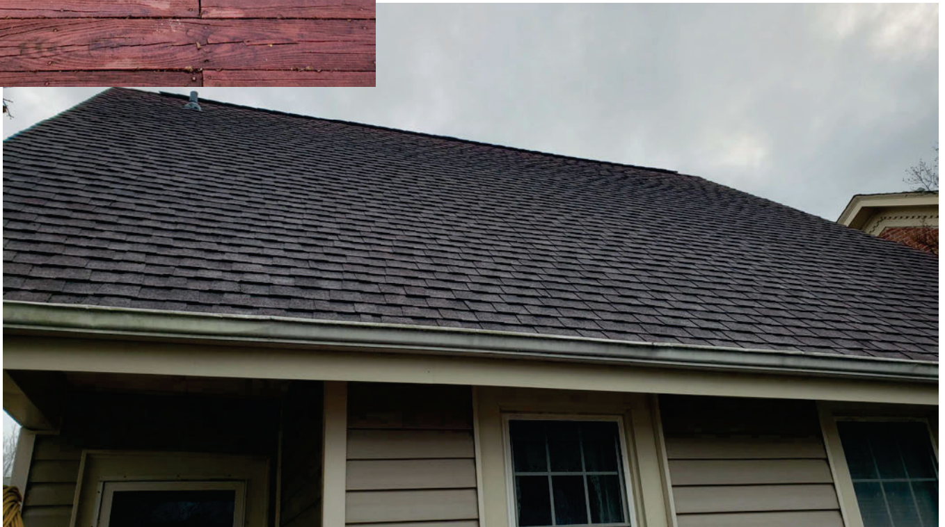
Back roof of 115 Randolph
