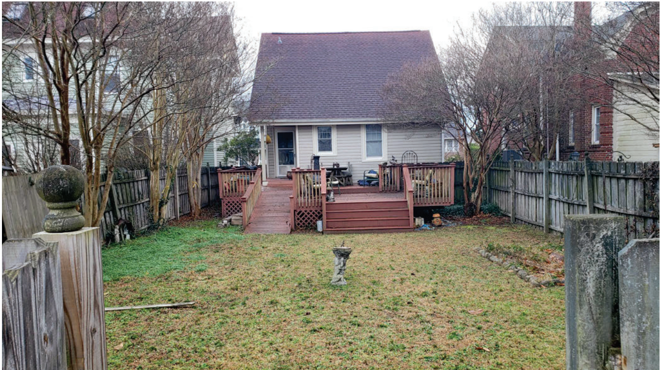
115 Randolph Ave current back of house, yard, fence, roof, deck, trees in both directions
