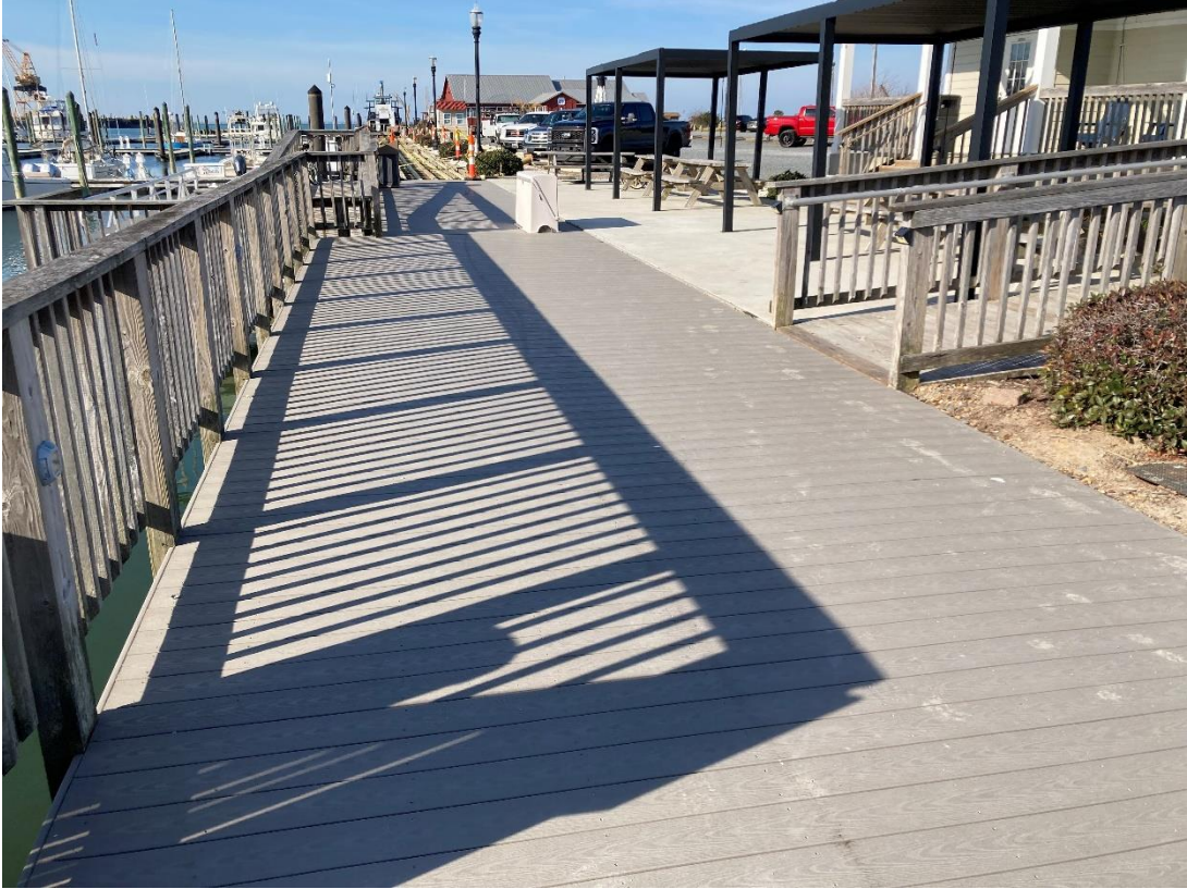
Phase 1 looking west and at northeast corner.
