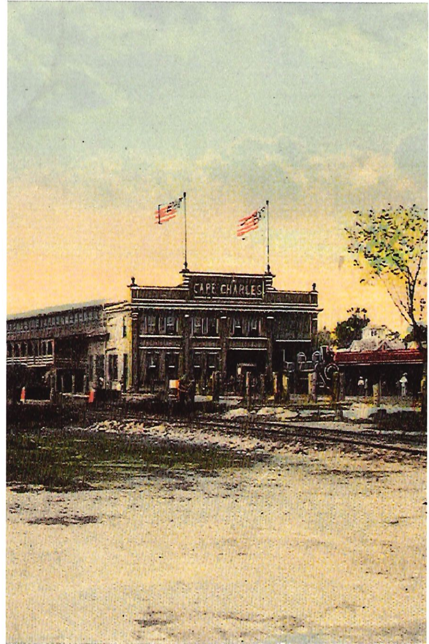
Cape Charles Harbor Terminal Building, 1911.
