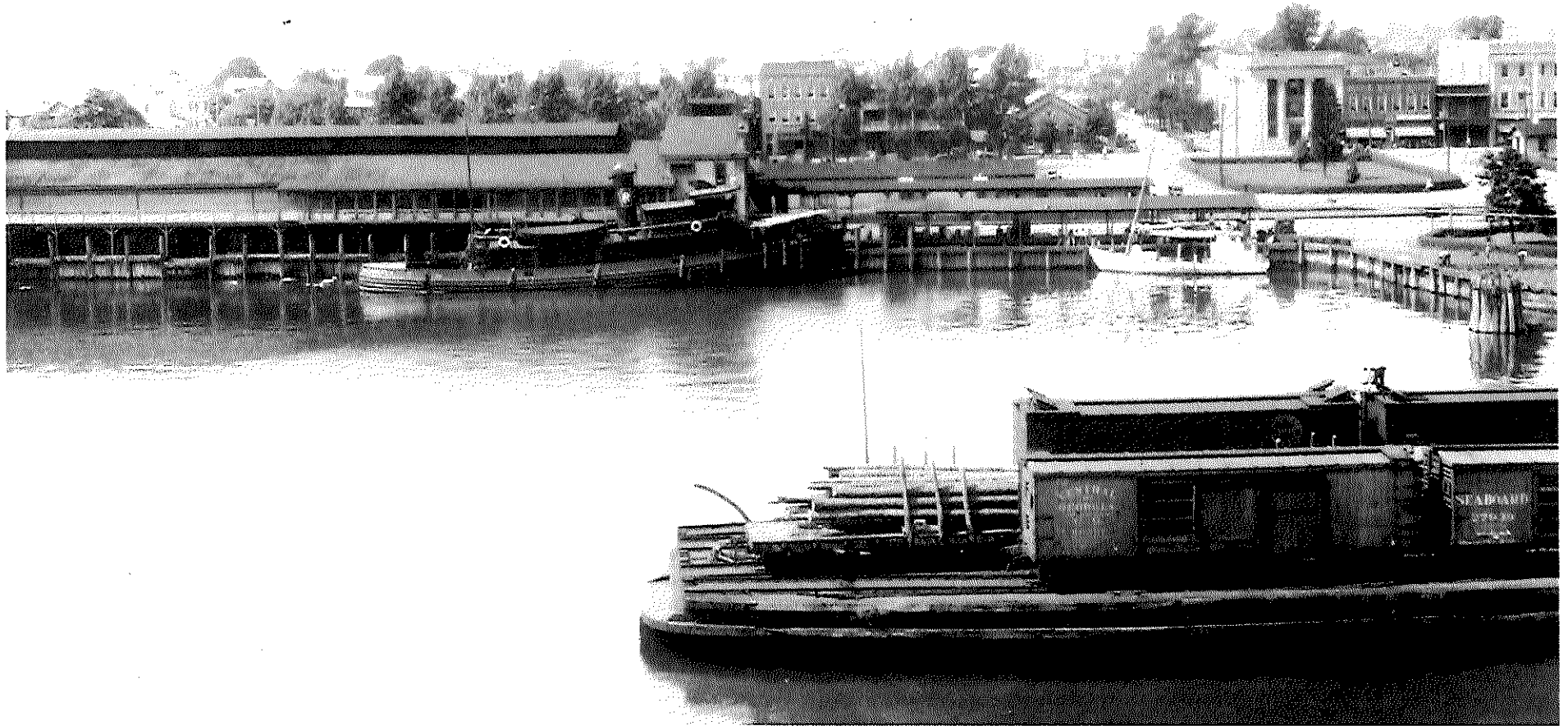
Image 2: Cape Charles Harbor and Monroe Ave, 1927. This view provides insight into the historic flow from the town across Mason Ave and into the railyard/harbor area. Public space extending from Pine Avenue functioned as a central axis. The axis and associated public parks and open spaces provided viewsheds and pedestrian access, with industrial-related structures built up along the harbor to the west, and along the railway to the east (see images 1, 5, and 11).
