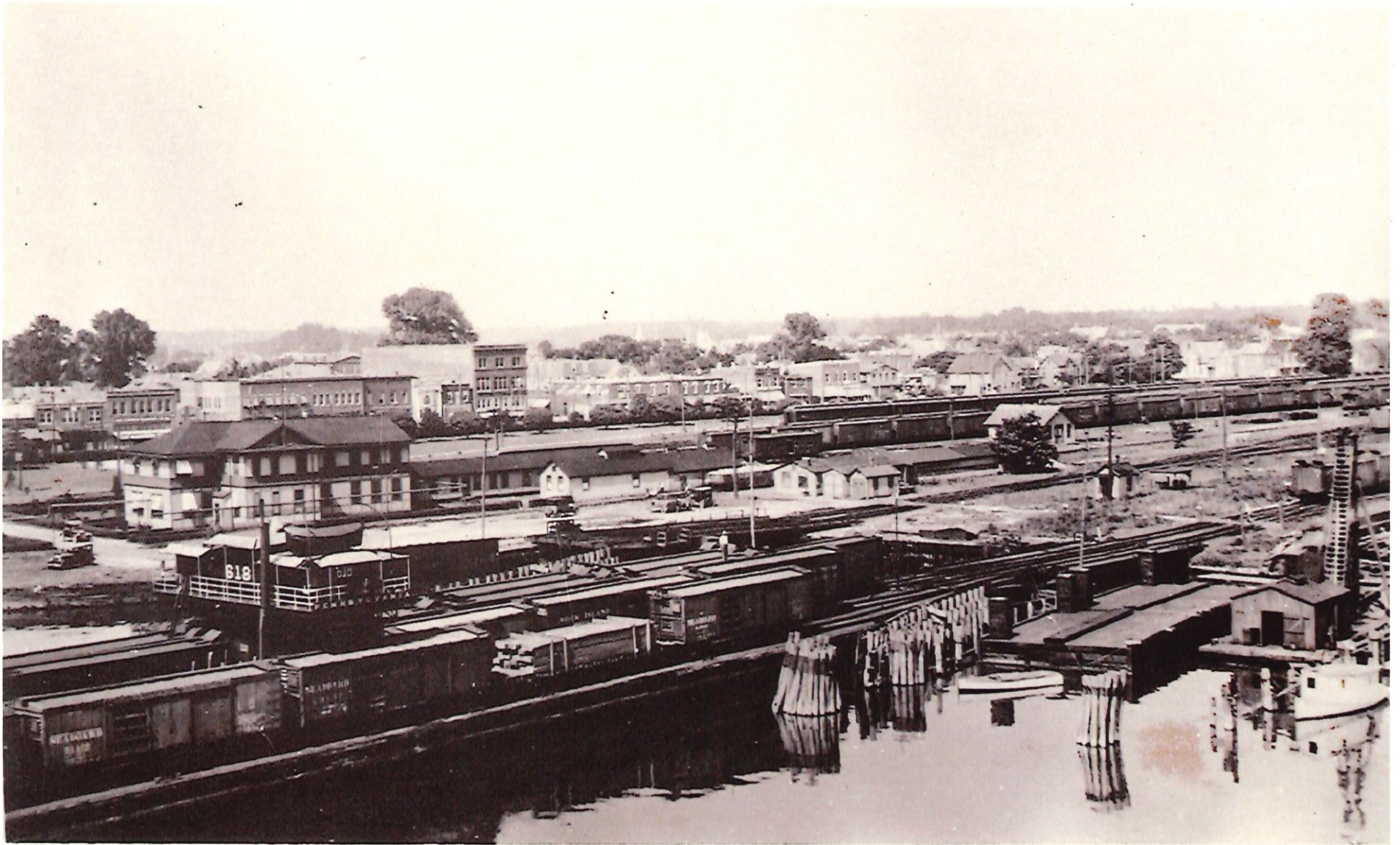
Image 12: Cape Charles Harbor and Railway, 1927. This view, looking east from the harbor, shows more of the Master Plan area, with Mason Avenue, green space, railways, and the harbor are all visible
