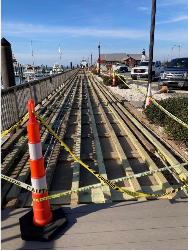
Phase 2 under construction looking west and east. Now completed.
