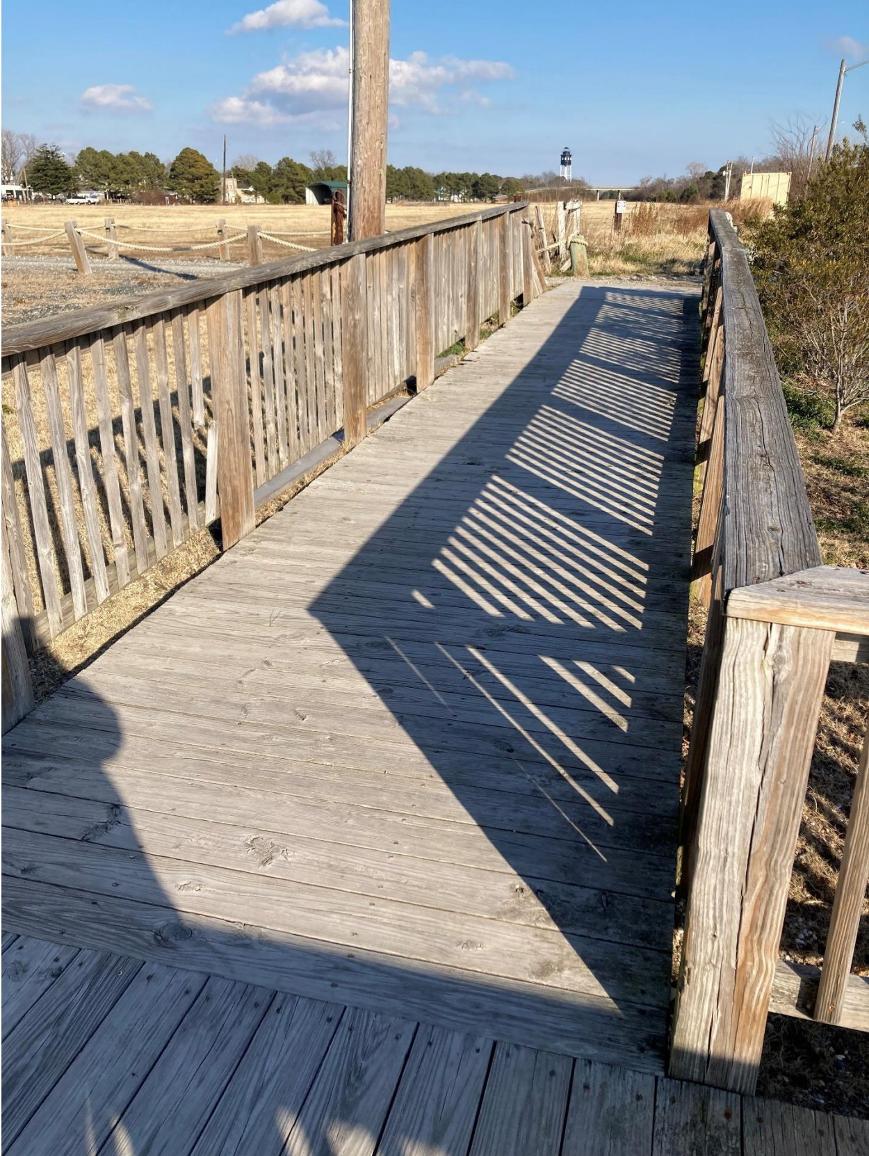
Phase 3 looking east.
