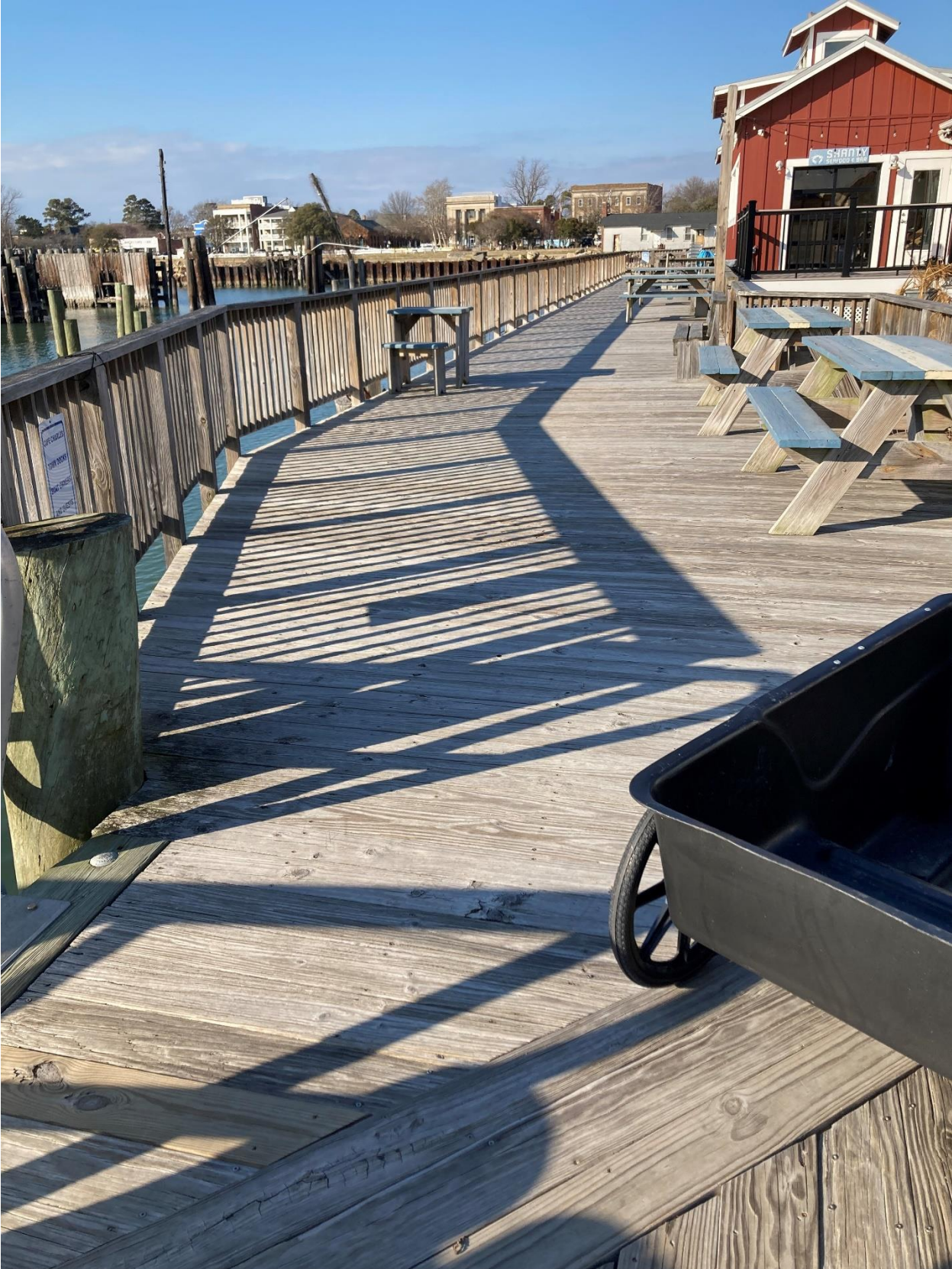
Phase 3 looking north.
