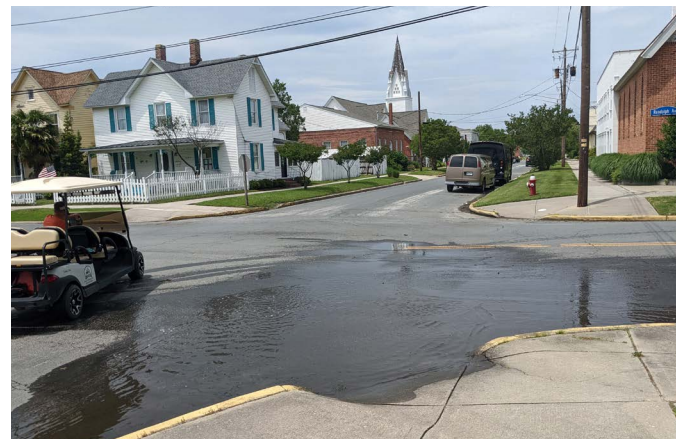
A golf cart drives past pooled stormwater.
