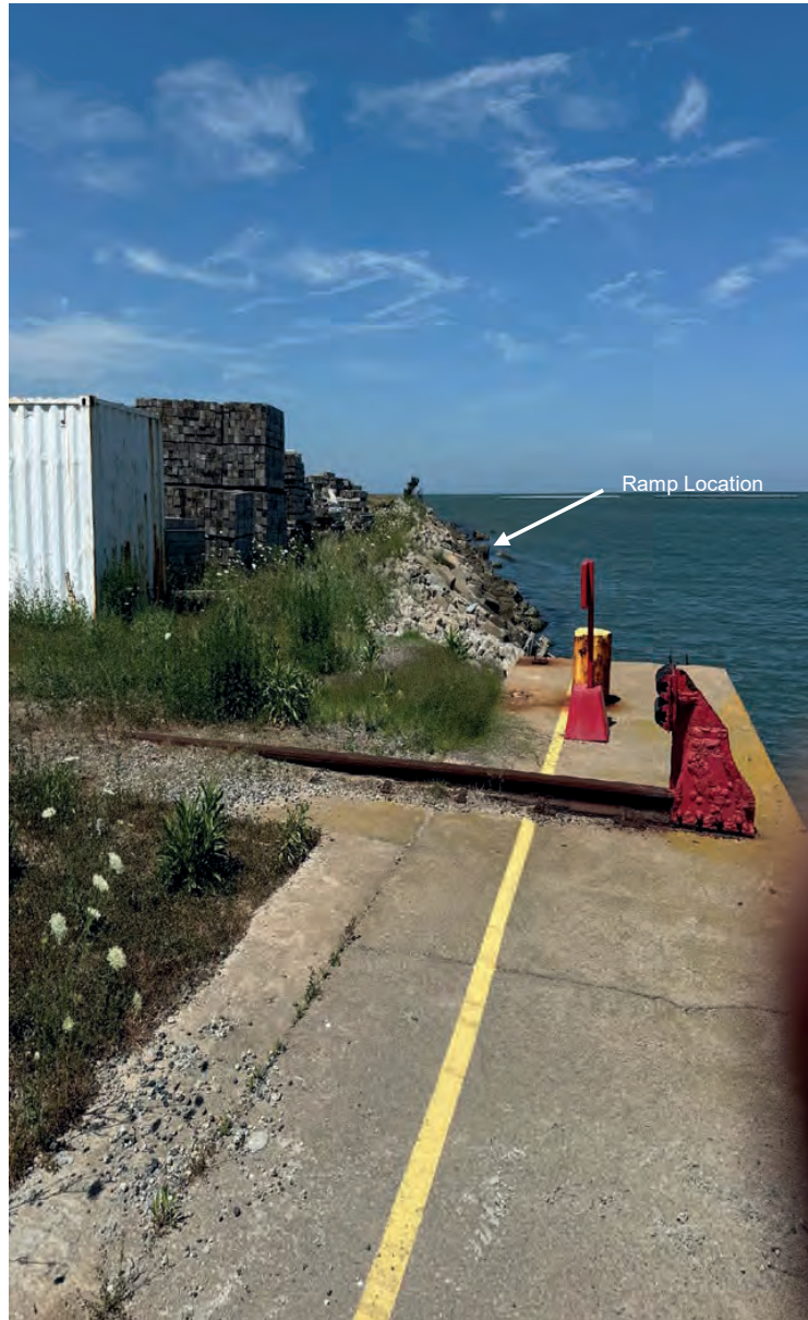
Photo 1 – Looking west along northern shoreline where proposed launch ramp would enter the harbor.
