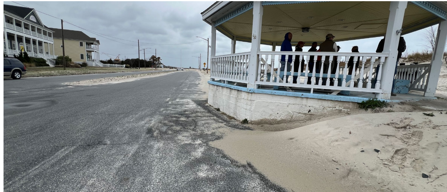
Windblown sand; the sand from the dunes is migrating past the Gazebo and into the road.
