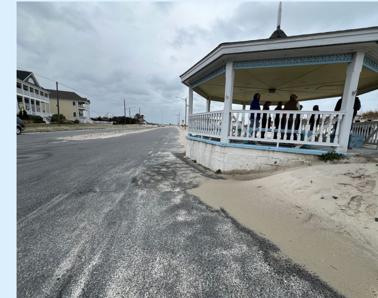
Windblown sand; the sand from the dunes is migrating past the Gazebo and into the road.
