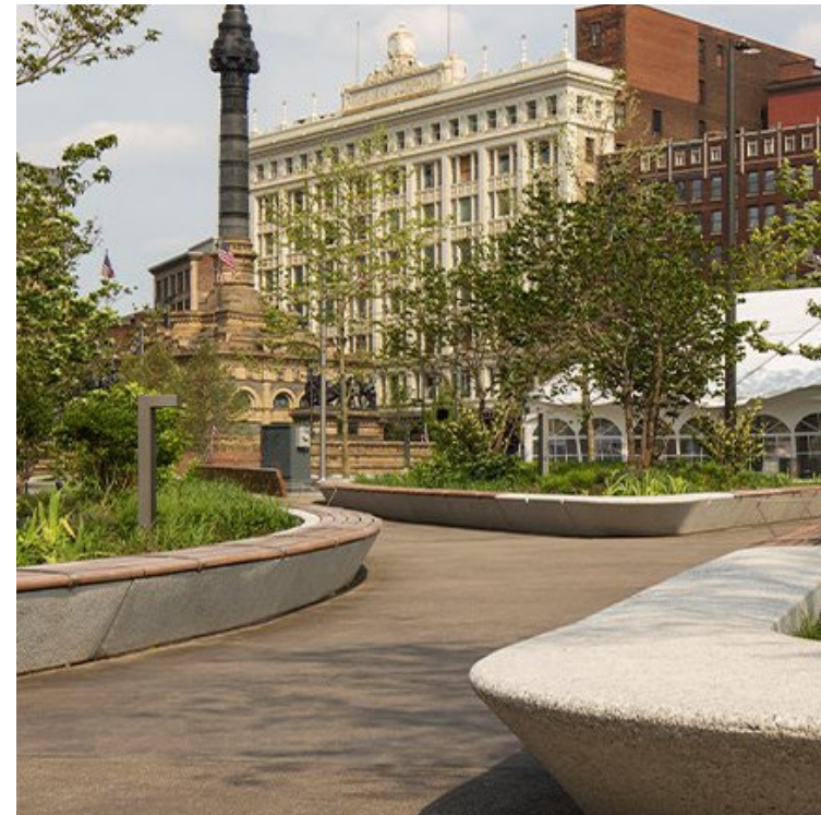
Cast in place concrete seat walls
