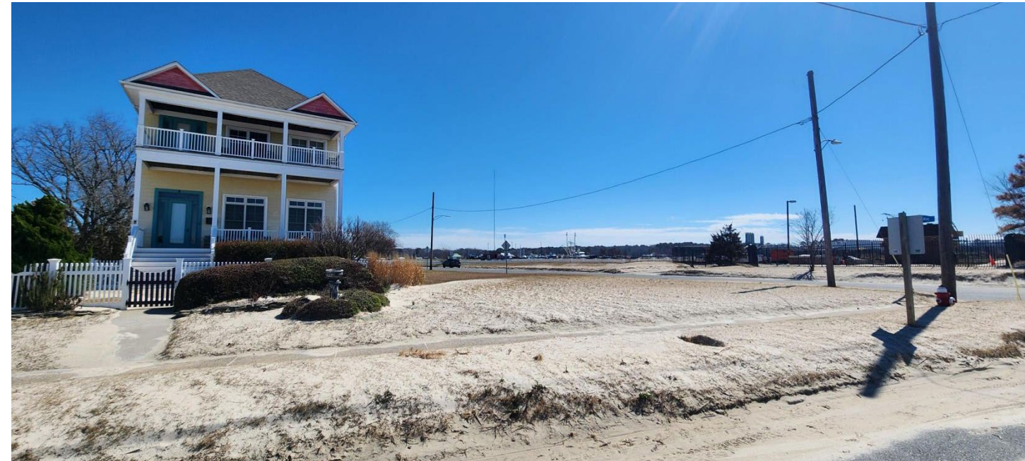
Existing Vegetation on dunes located along Bay Avenue
