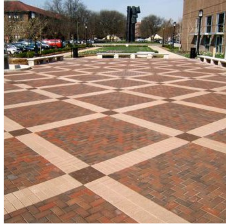
Cross Pattern Brick Paving
