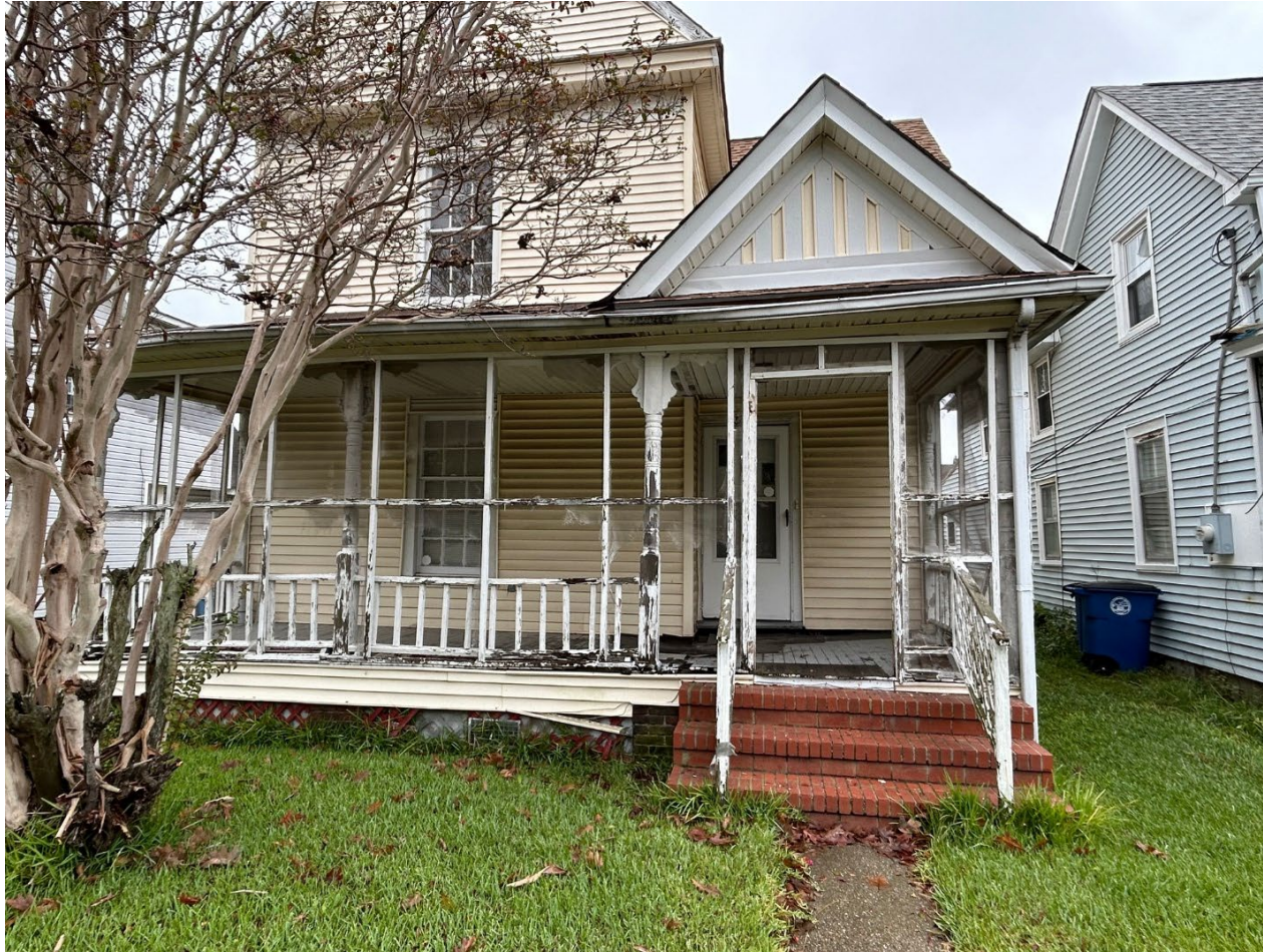
537 Mason Avenue Existing Conditions
