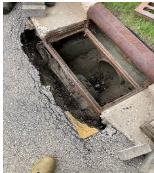
Repaired all storm sewer inlets in Chestnut Grove
