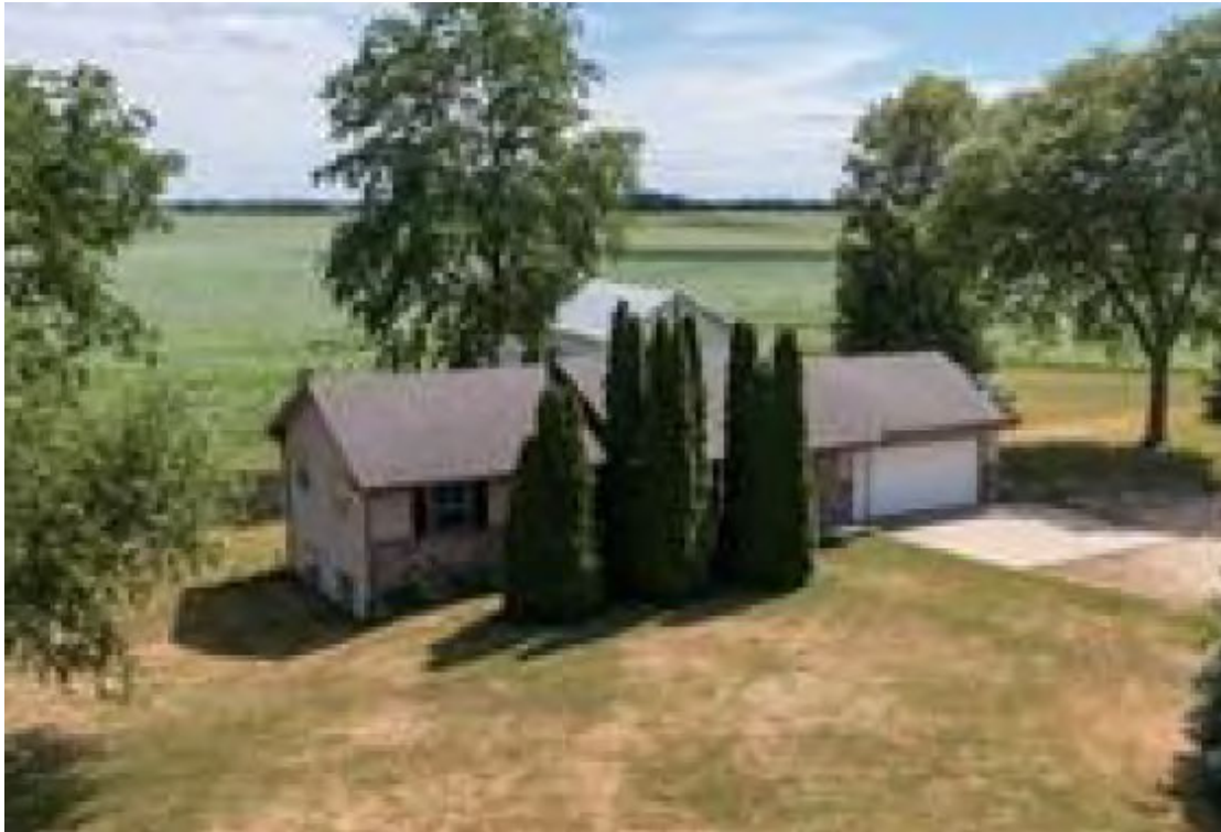
8010 Trask Bridge Road, Rockford, IL
