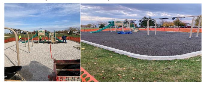
• Removed pea gravel from Suppeland Park tot lot, refilled area with crushed stone, and installed safety surface.
