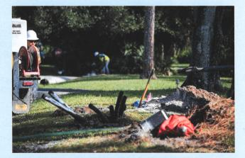
directional boring or horizontal directional drilling, installs underground piping to safely place our electric cable to connect power to your home or business. Unlike open trenching, directional boring allows FPL to install underground equipment while minimizing impact to trees and other vegetation on your property. The underground facilities will be installed 36 inches to 48 inches below the surface, or deeper, if necessary, to avoid tree roots.
