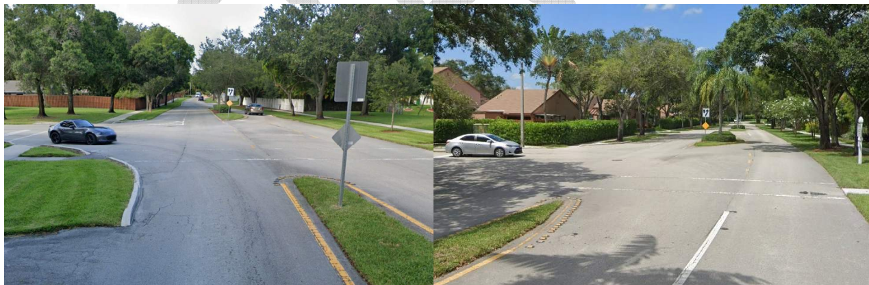
Figure 41 Stonebridge Pkwy. Uncontrolled Marked Crosswalks at W Lake Blvd. and N. Lake Blvd. looking northeast respectively.
