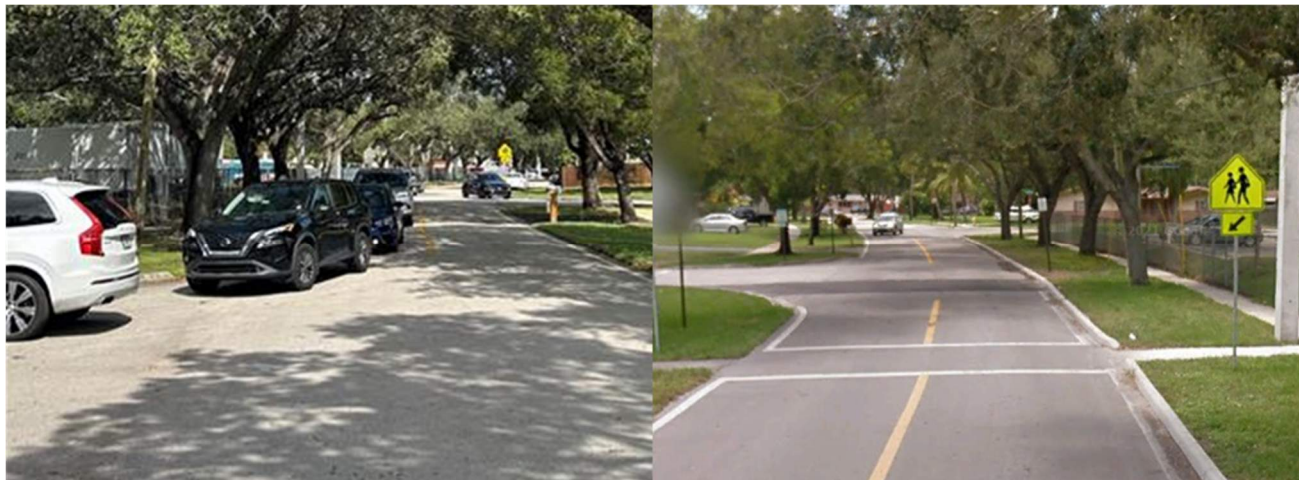
Figure 31 SW 51st St. at SW 92nd Ave. looking east and uncontrolled marked crosswalk north of SW 91st Ave. respectively.
