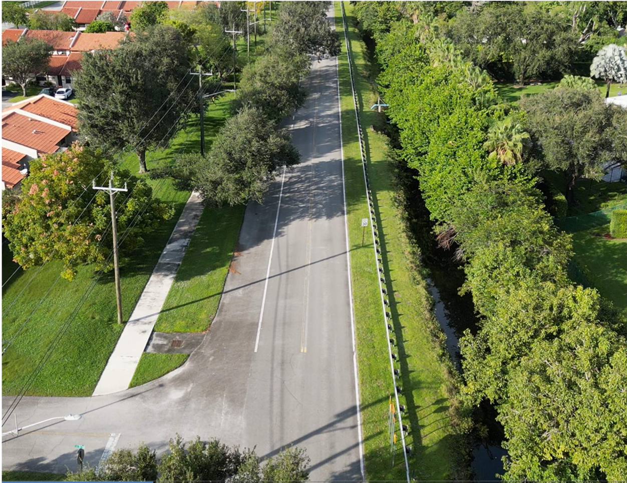
Figure 25 Hiatus Rd. at SW 57th Cir. looking north.
