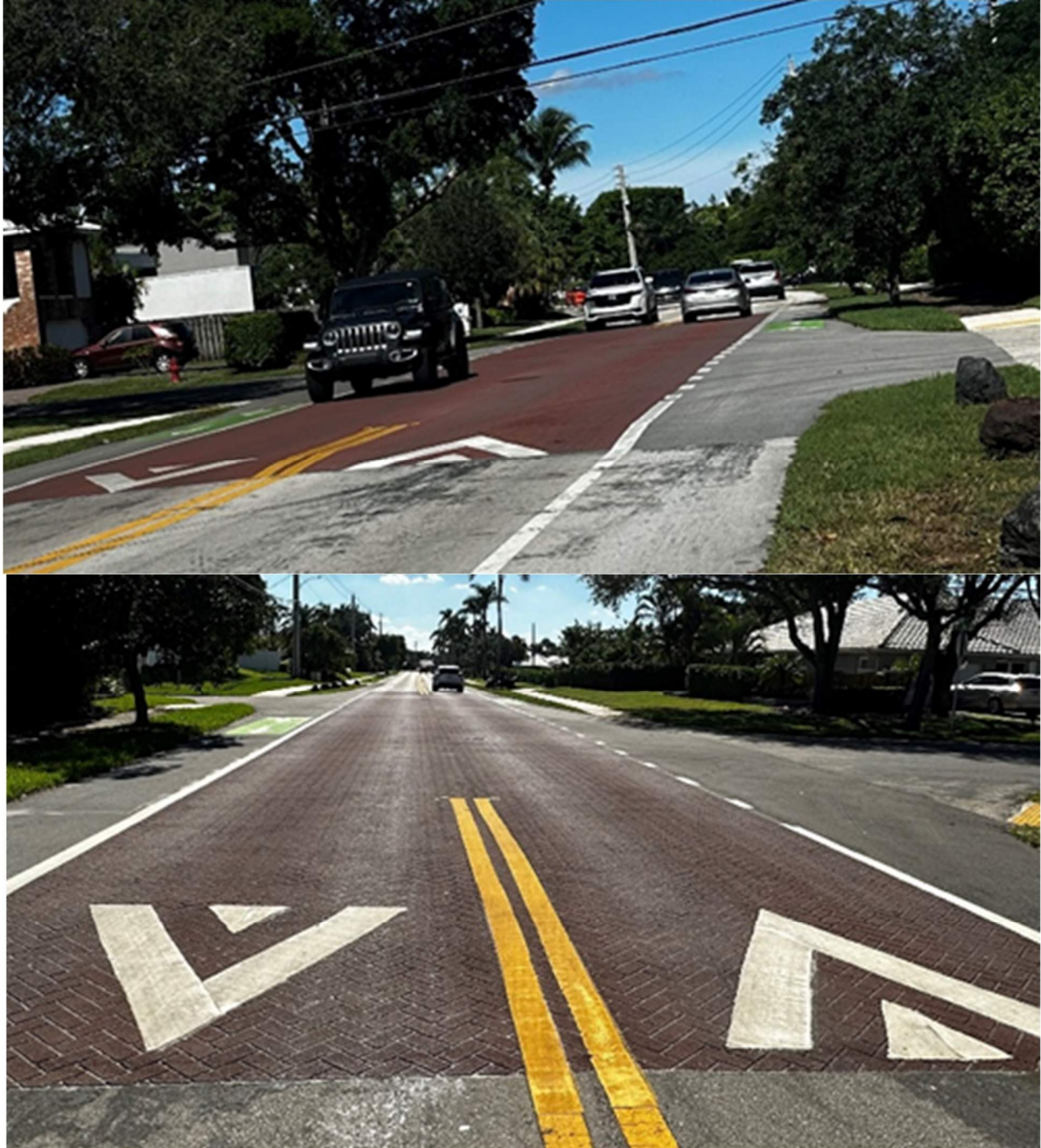
Figure 43 Images of speed tables with texture pavement through intersections within Broward County.
