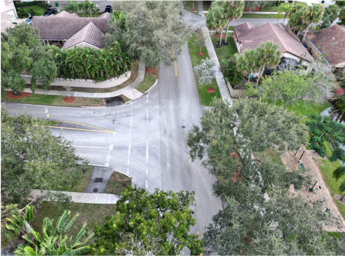
Figure 34 Stonebridge Pkwy and NE Lake Blvd. looking south.
