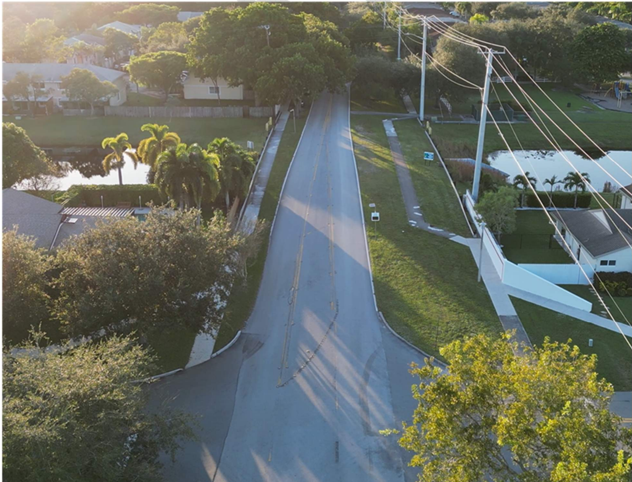
Figure 18 SW 49 th St. at SW 120 th St. looking west.
