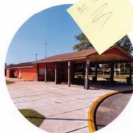
3. ORANGE PAINT & ASPHALT SHINGLE ROOF
