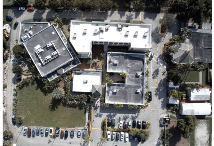
Nur-UI-Islam parking lot was able to satisfy the parking demand during the afternoon service of the Mosque
