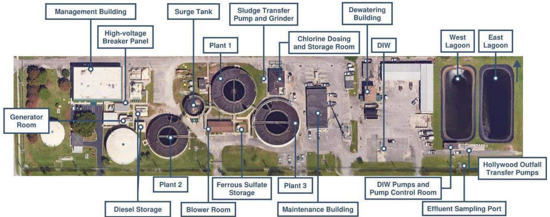
Figure 2-3: Existing WWTP Site Aerial
