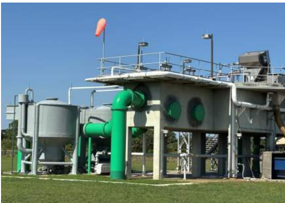
City of Port St. Lucie Glades WWTP Screening and Grit Facility
