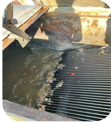
Manual Bar Screen at Surge Tank and Treatment Units
