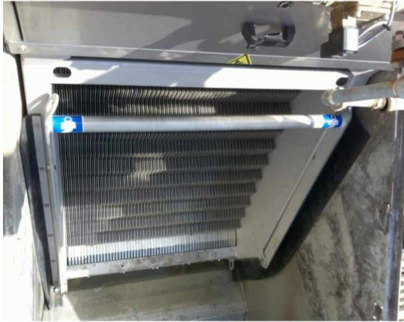
Figure 4-3: Step Screen (courtesy of Huber Technology)
