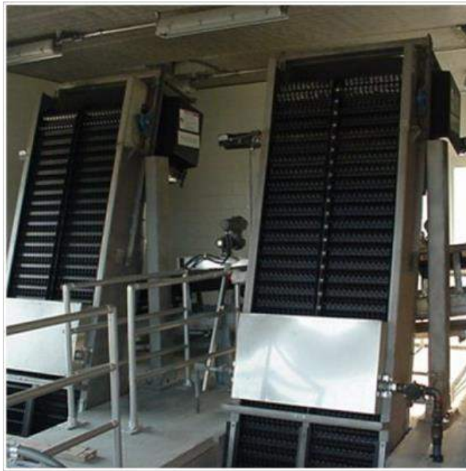
Figure 4-4: Continuous Belt Screen (courtesy of Parkson Corporation)
