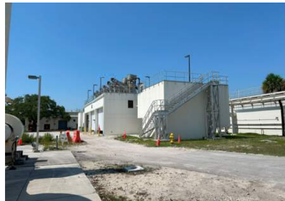
Broward NRWWTP Grit Structure and Grit Building
