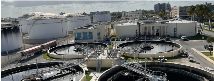
Figure 6.1. Fort Lauderdale MCC Replacement at GTL WWTP
