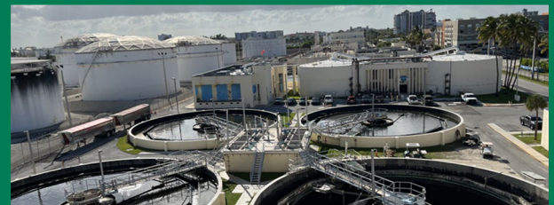
Figure 5.5. Fort Lauderdale MCC Replacement at GTL WWTP
