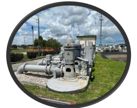
Transfer Pumps to SRWWTP
