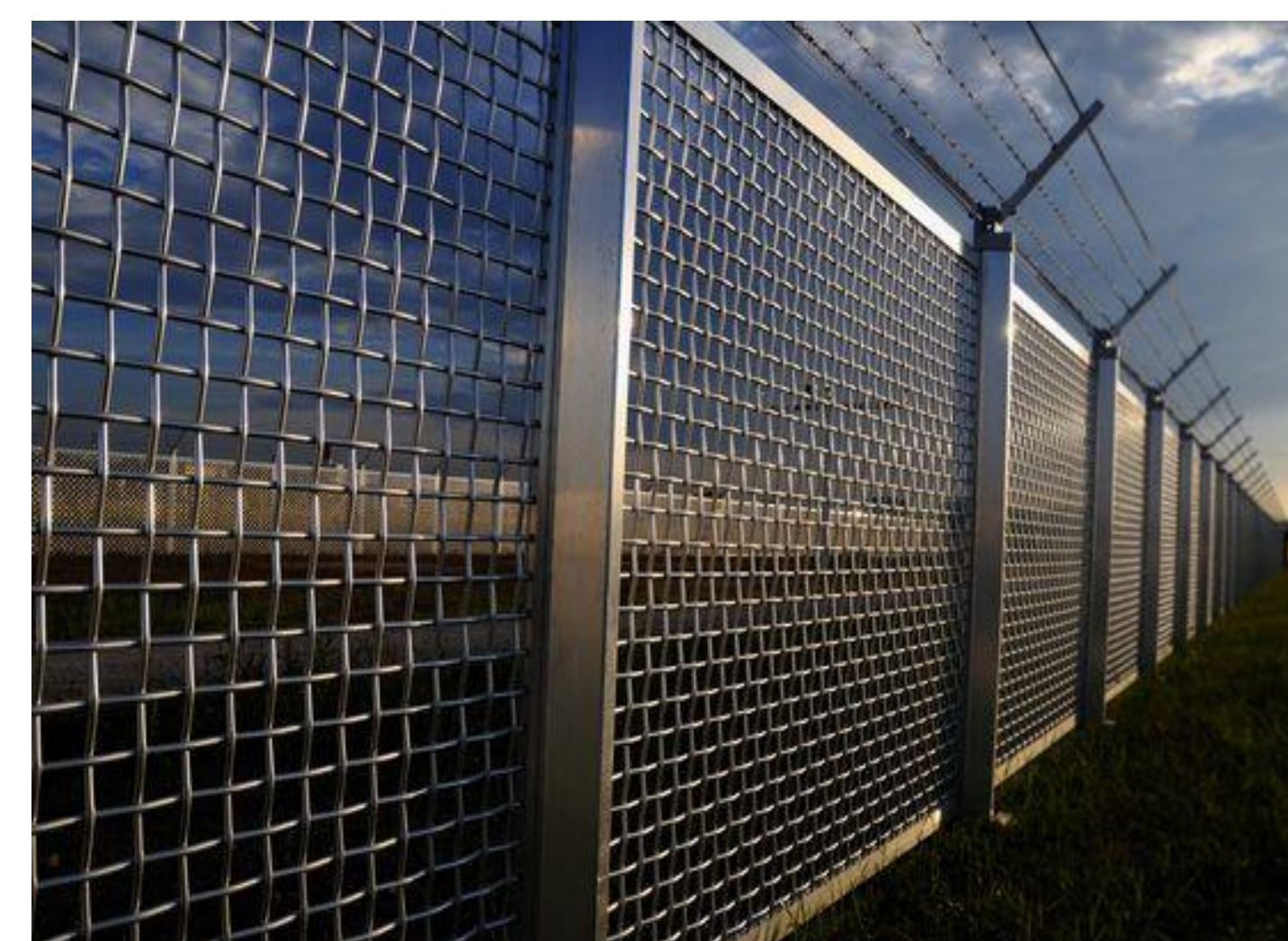
Perimeter Fence Type C
