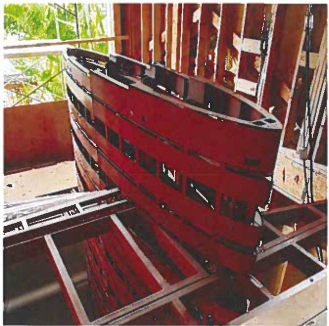
A solid stair structure to be clad in stone and wood for private residence in Hawaii. Case Study >>
