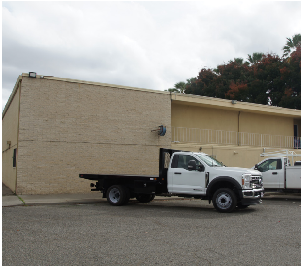
Figure 1.20: Image indicates existing empty wall on Riverside Inn on 5th Street.
