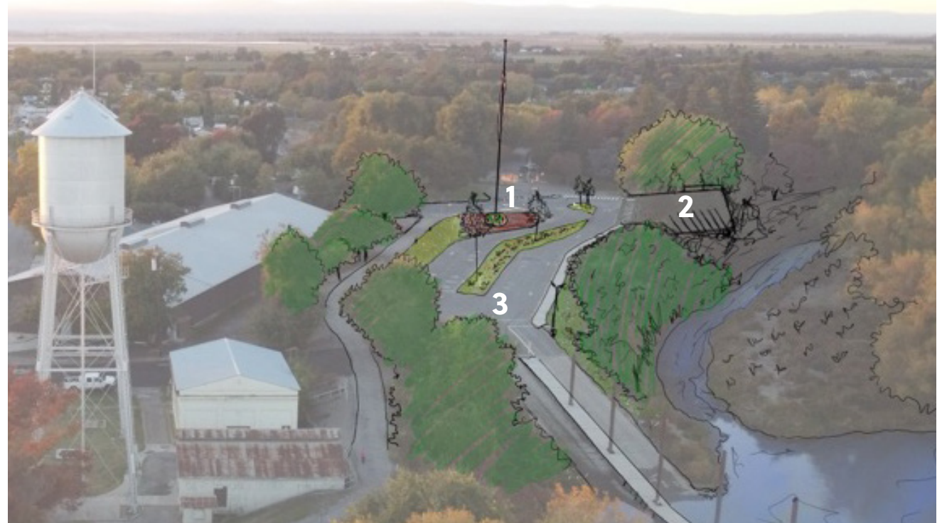
Figure 3.10: Boat Ramp Area
