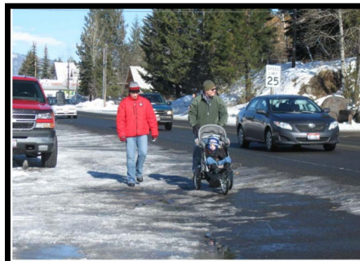
Pedestrians navigating a portion of the existing SH55 corridor without sidewalk.
